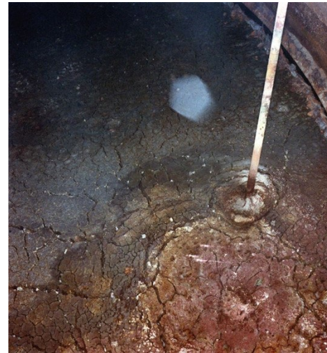
Sludge – 12 million gallons
