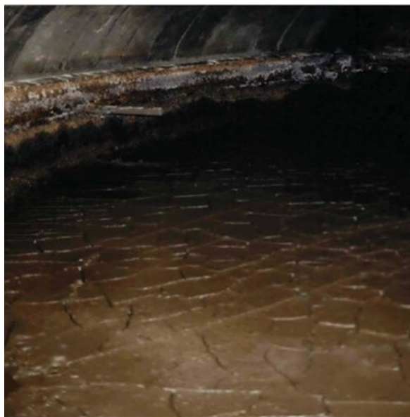
Sludge – Tank T-111
