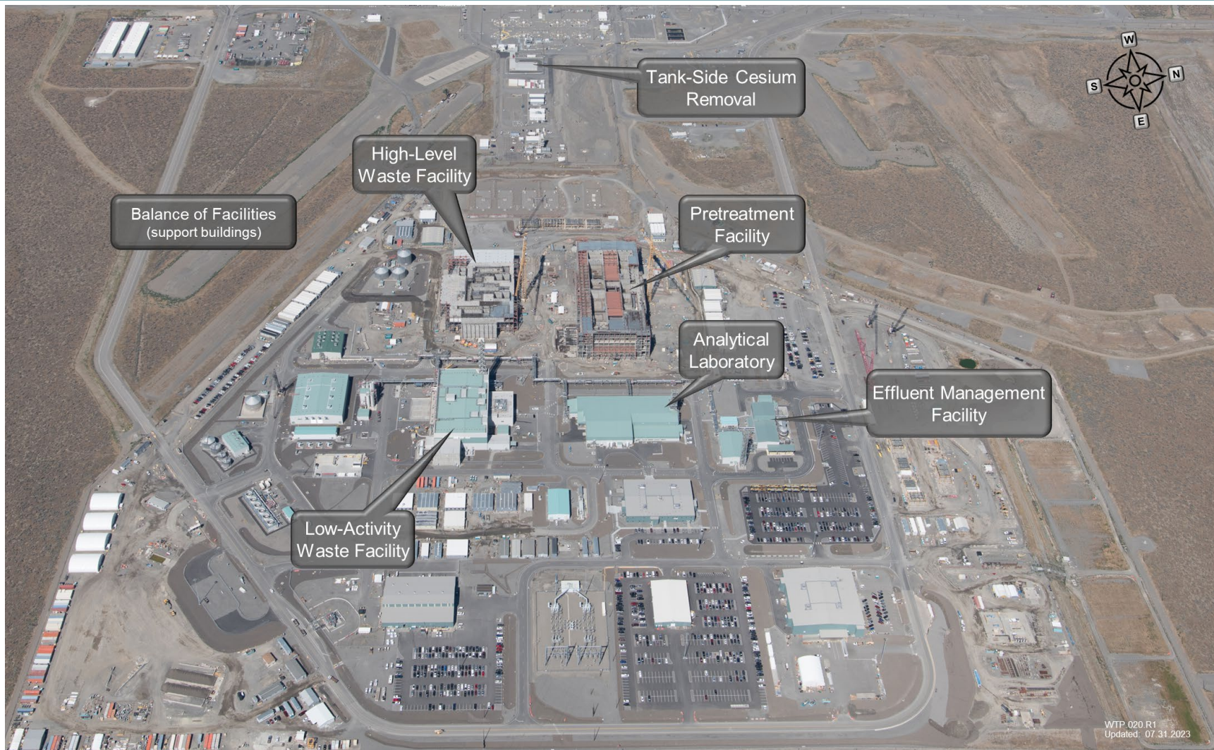
Aerial photograph of WTP facing west taken June 2022.
