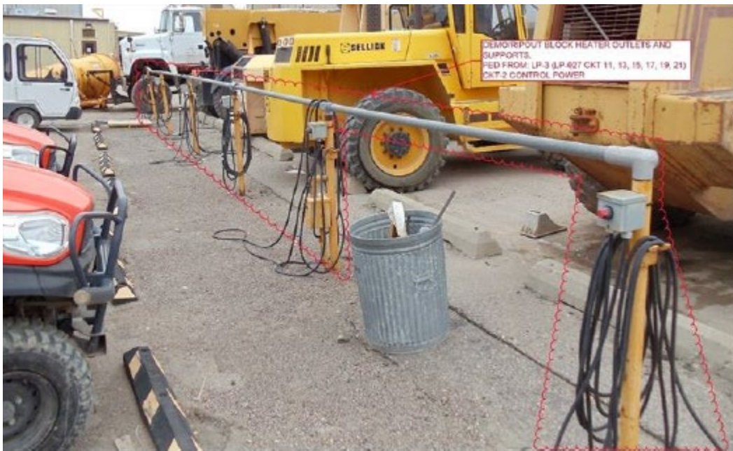
Block Heater Outlets for Vehicles
