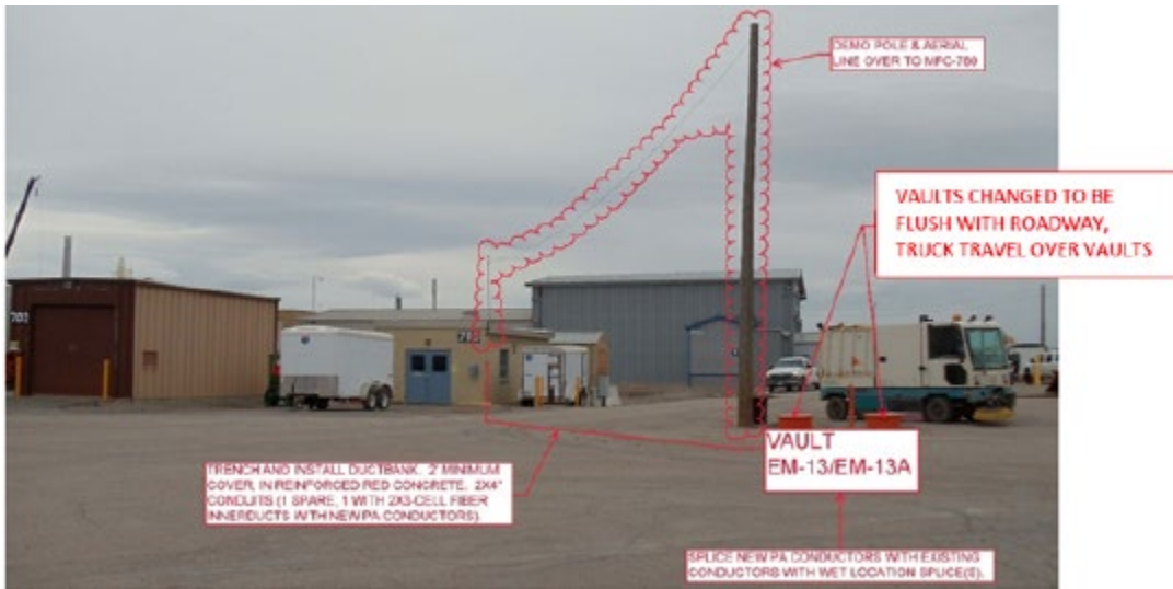
Power Pole to be Removed, Aerial Lines Re-Routed
