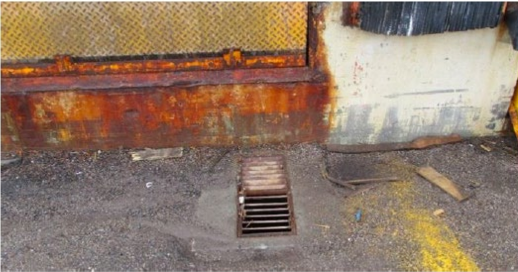
Drainage Inlet in Middle of Dock
