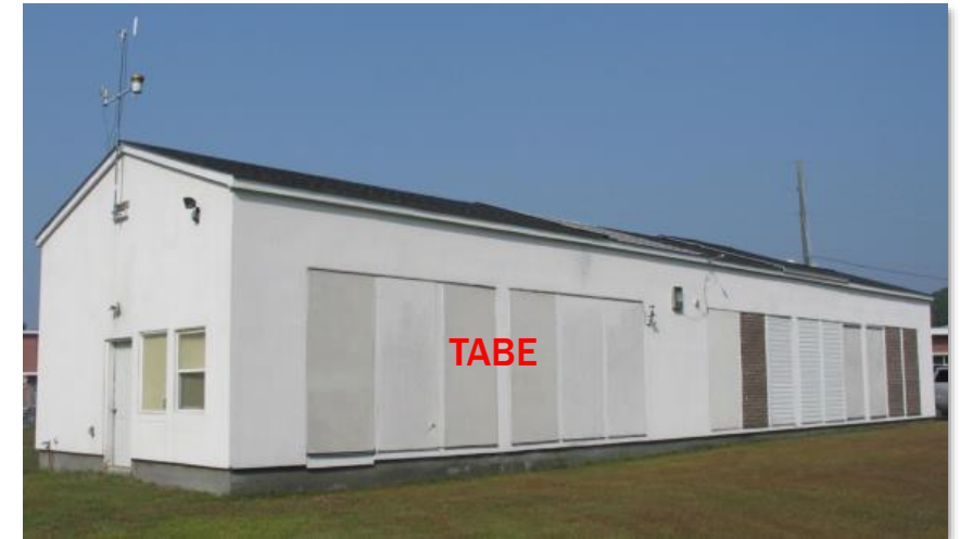
NET facility at Charleston, SC. Four wall panels in this NET facility are TUBEs.
