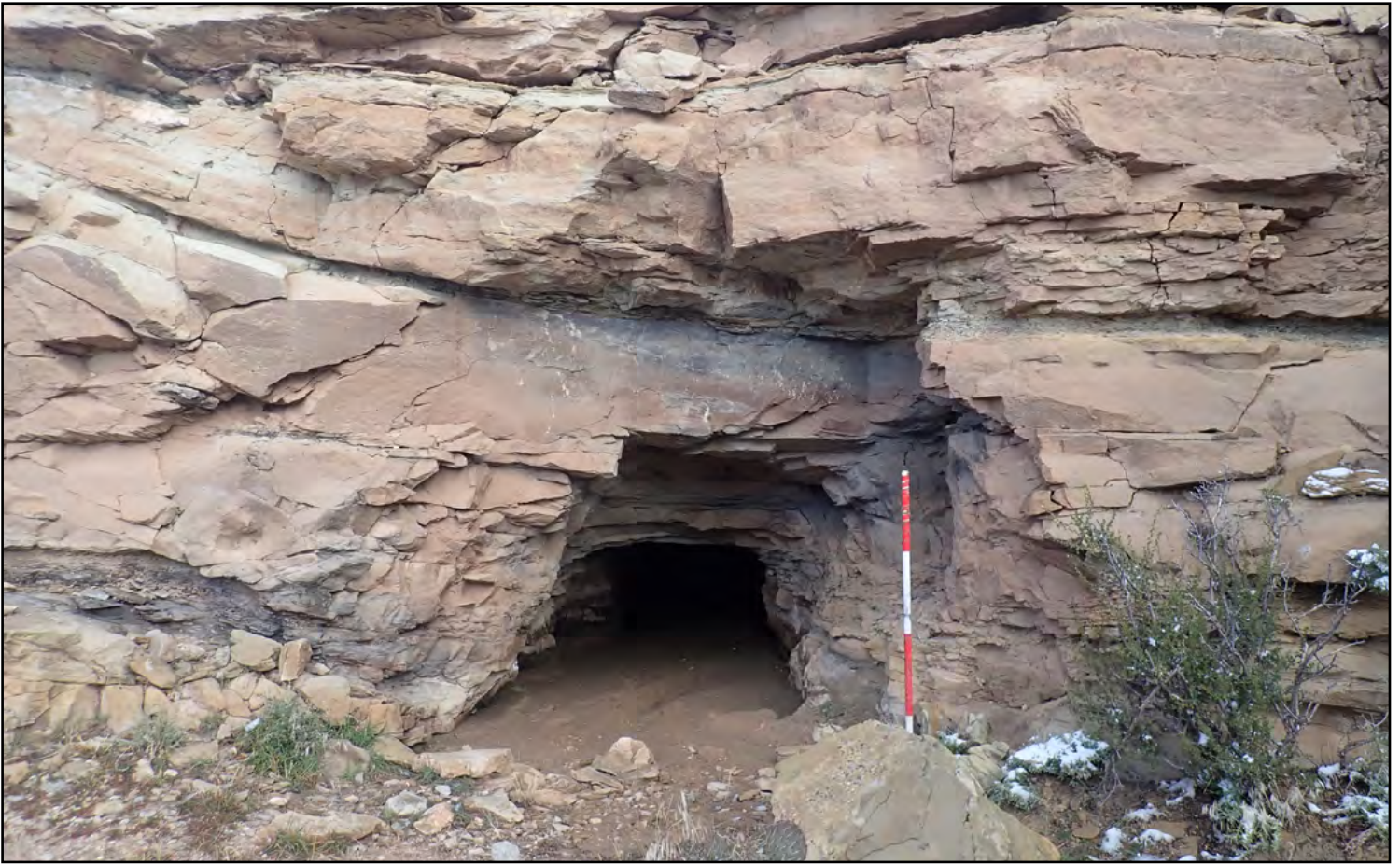
Open adit at the School Boy mine where the DRUM field team noted standing water 20 feet inside the adit.
