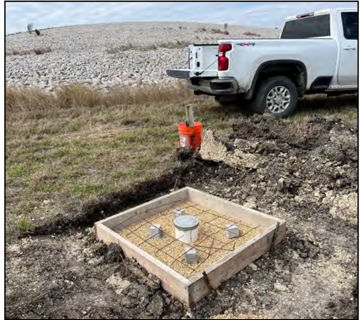
The form built for a quality-control monument before concrete was poured.
