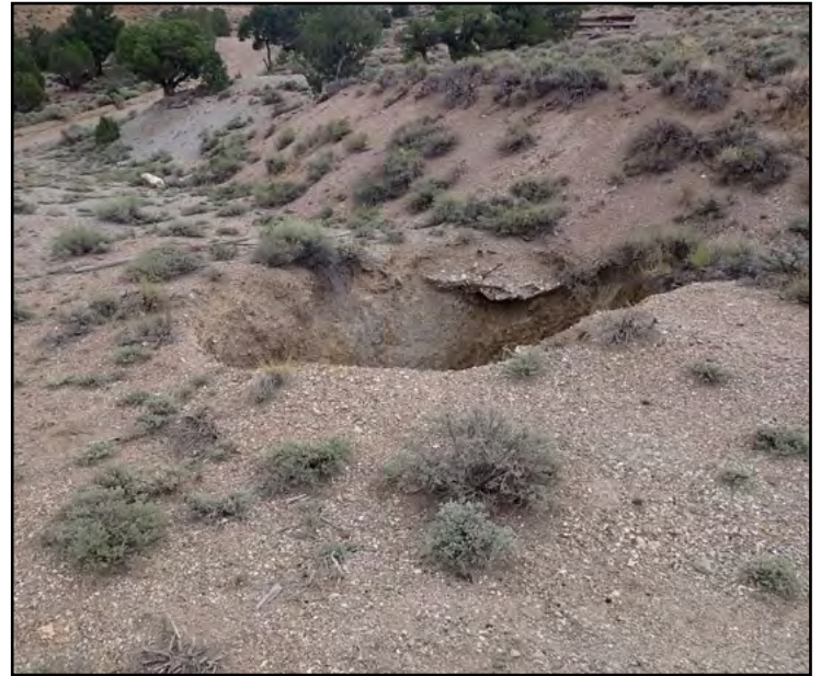
An open shaft at a DRUM site near Marysville, Utah.
