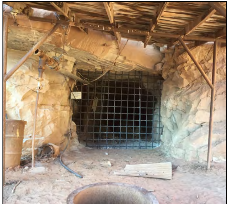
Closed adit at a DRUM site in White Canyon, Utah.
