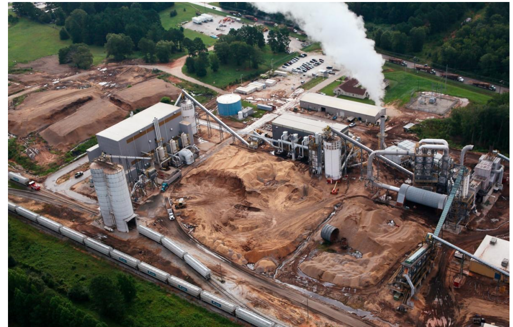
Enviva Biomass plant in Greenwood, SC, Southwings@ViewsfromAbove
