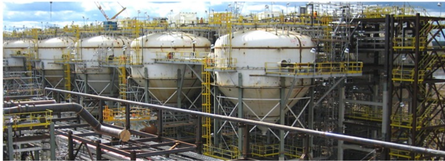
INCLINED PLATE SEPARATORS UNDER CONSTRUCTION AT THE HORIZON FROTH TREATMENT FACILITY (PHOTO COURTESY CANADIAN NATURAL RESOURCES)
