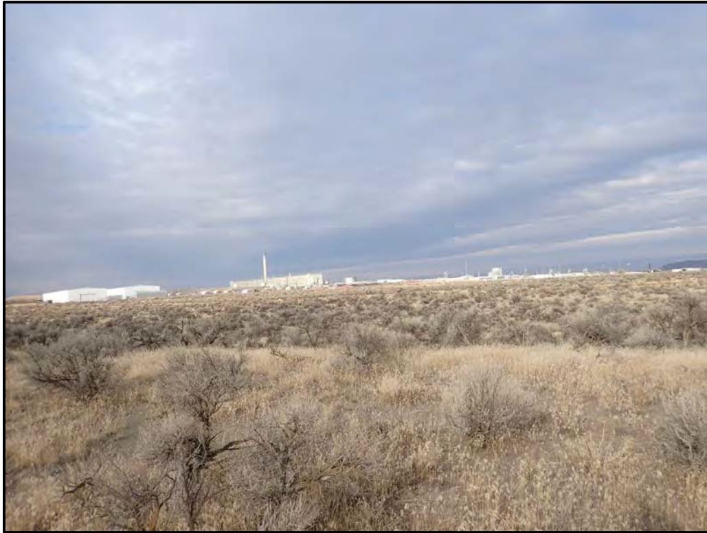
Figure 6 – Overview of South Construction Support Area
