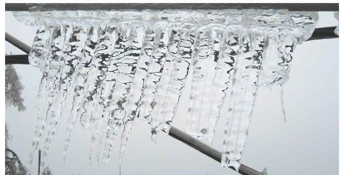
The accumulation of ice on utility lines can cause damage that may result in power outages.
