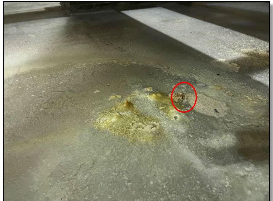
Remnants of missing plug below wet decon pump
