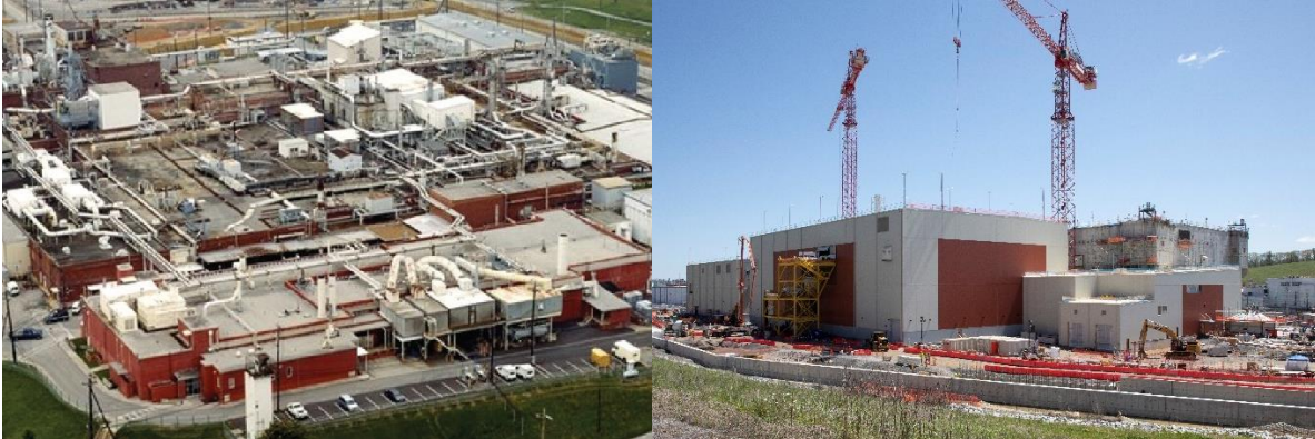
Manhattan Project-era Building 9212 at Y-12 (left) and construction on its replacement, the Uranium Processing Facility, in April 2022 (right)
