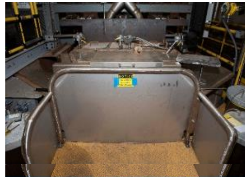
Restored electrolytic cell at Y-12
