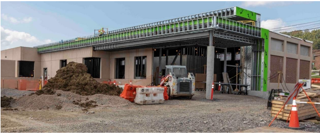
Construction at the Emergency Operations Center at Y-12
