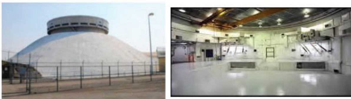
Figure 4. INL ZPPR cell. Outside view (left) and inside view (right).
