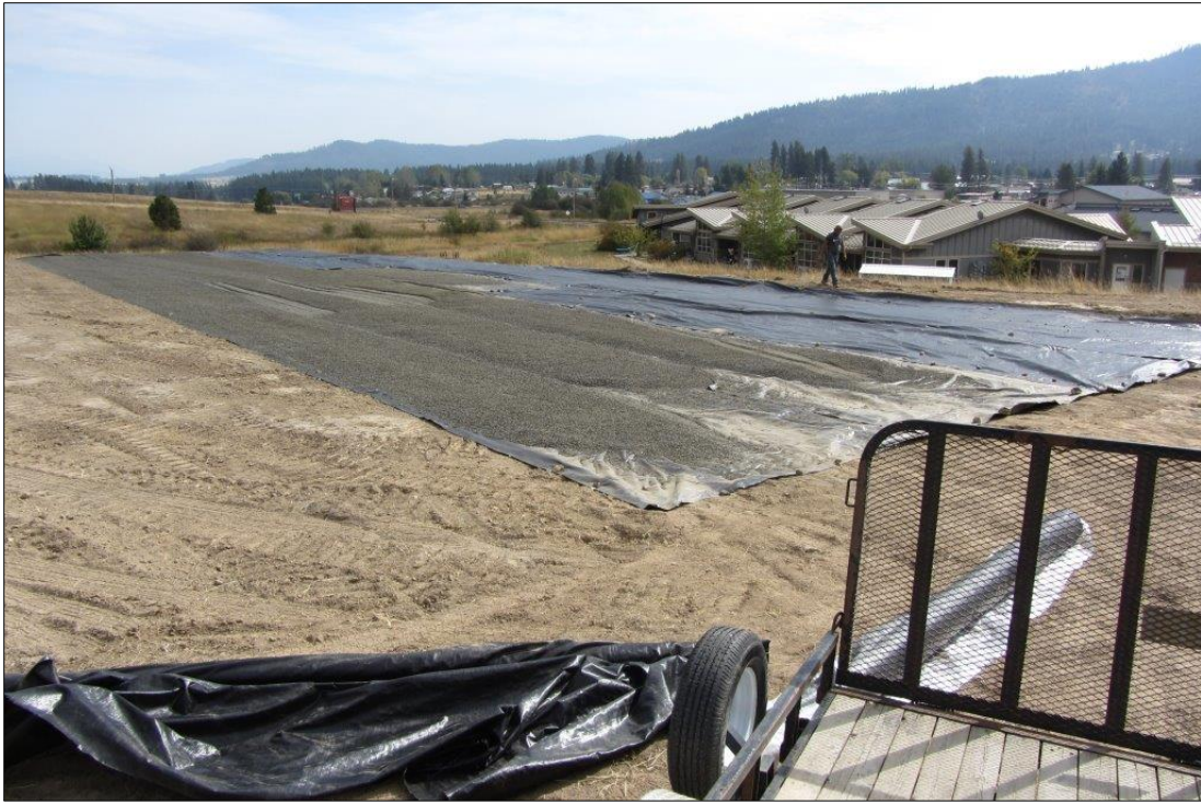
Site Preparation with Grading, Fabric and Rock
