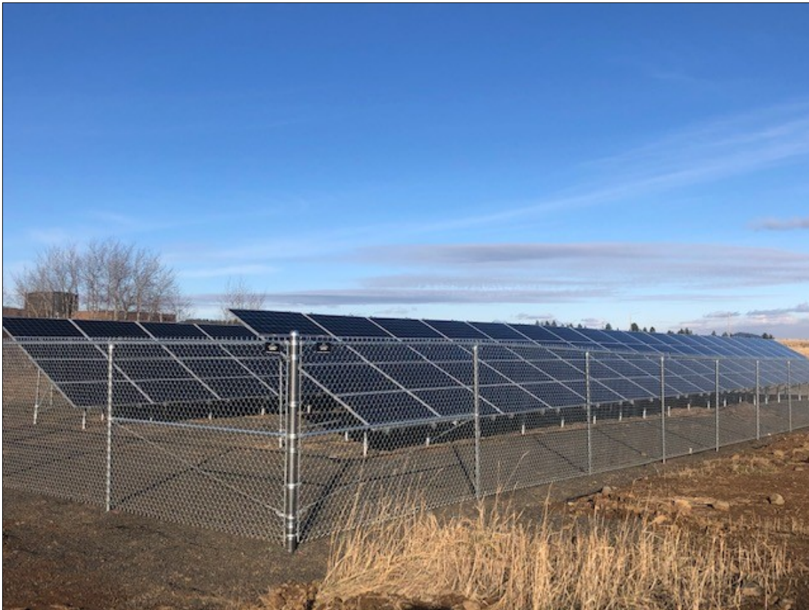
Completed Solar Panel Installation
