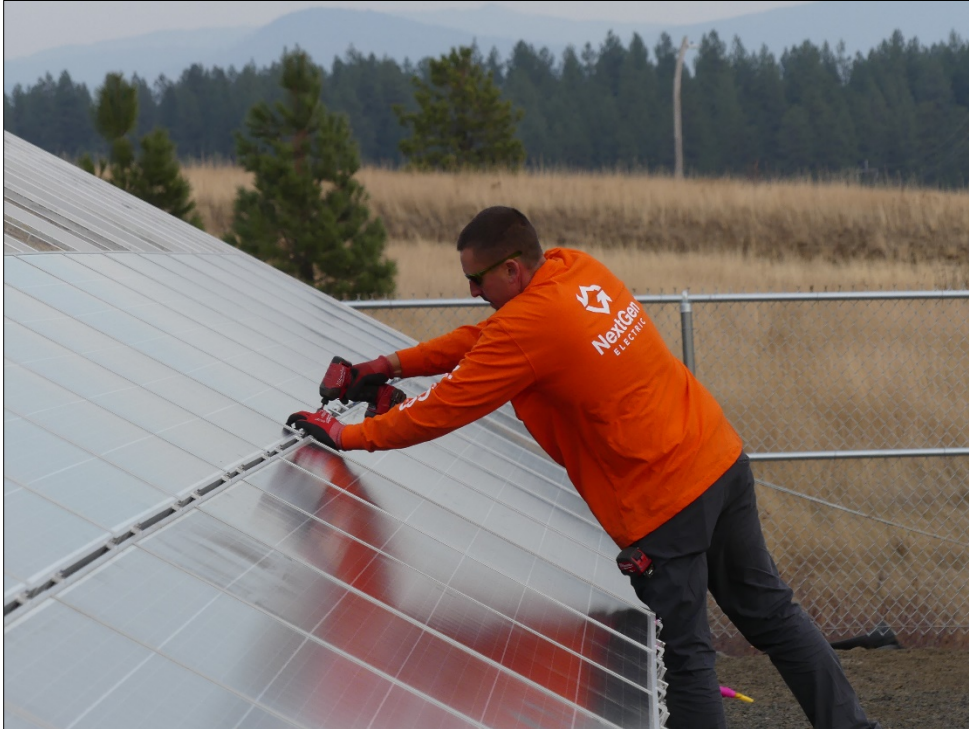
Installing Solar Panels
