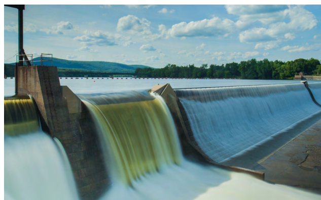
A General Electric Research-led team demonstrated a new hydropower turbine design and monitoring methodology that allows plant operators to adjust power output in a few seconds to meet energy demand without needing to start or stop units. Image from American Public Power Association, Unsplash
