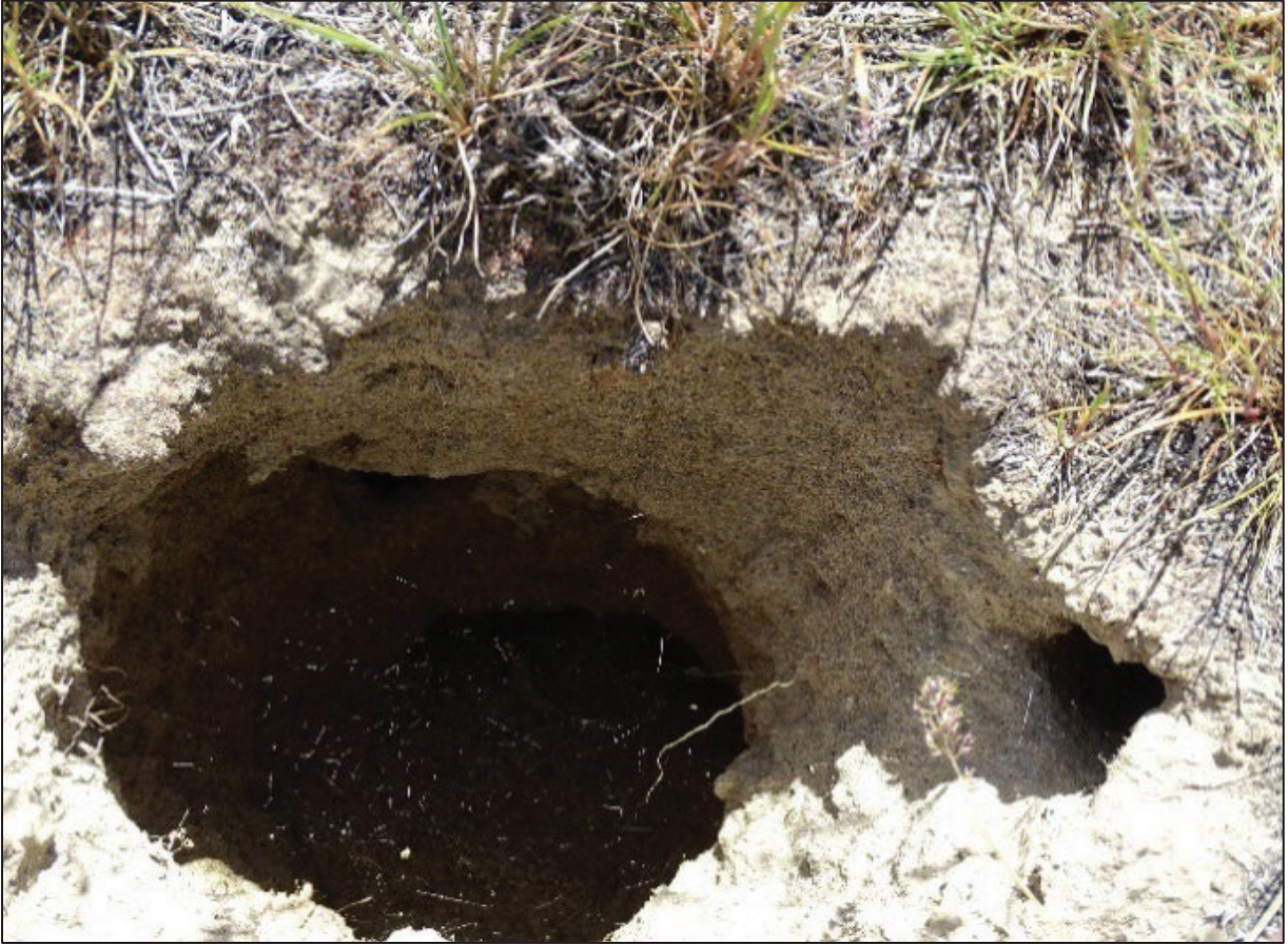
Figure 1. Sinkholes and Subsidence Areas at Nike Missile Launch Site H-12-L (WIDS 600-6)
