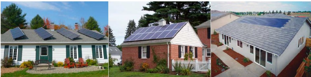
Least integrated (Open rack-mounted PV)
