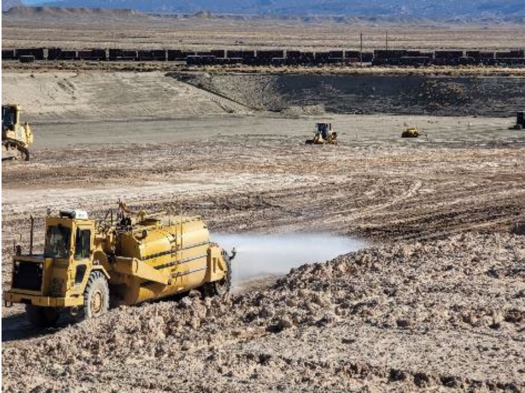
Photo 11. Moisture Conditioning RRM November 2021
