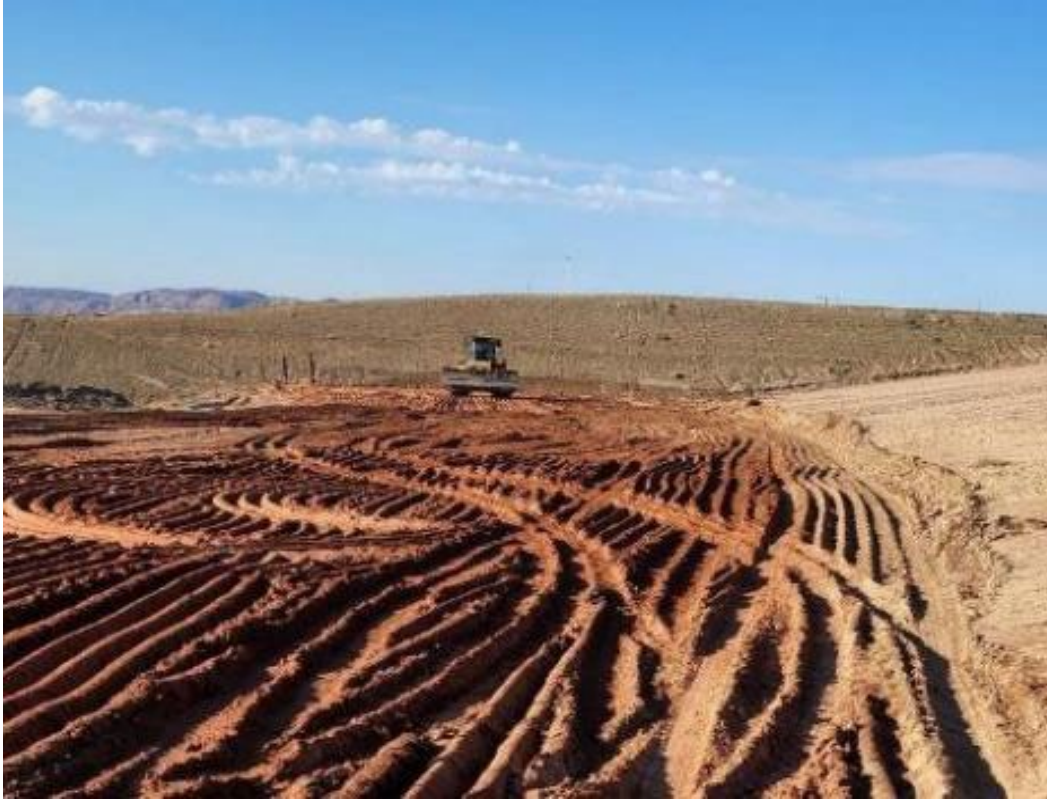
Photo 55. Compacting Looking South July 2022
