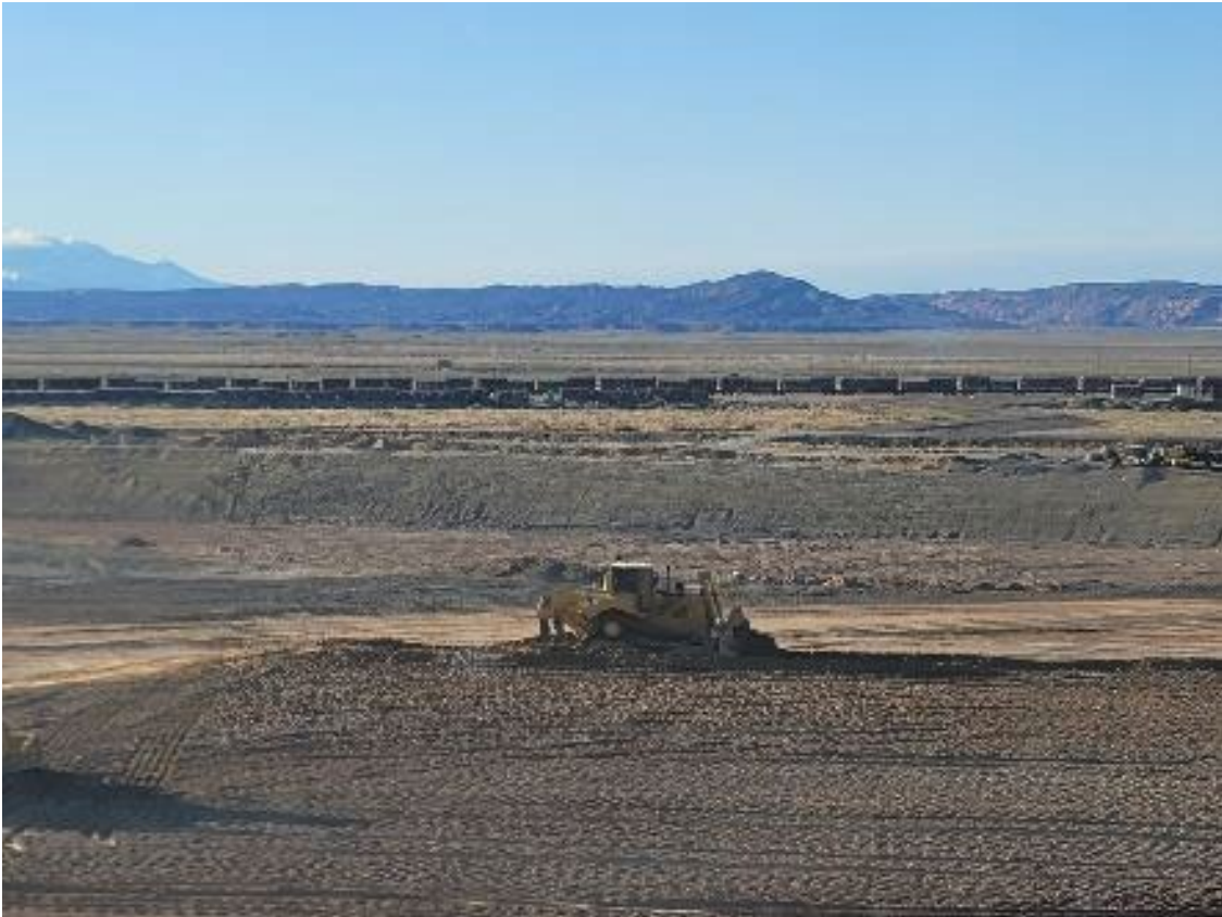
Photo 41. Pushing RRM on Lift April 2022
