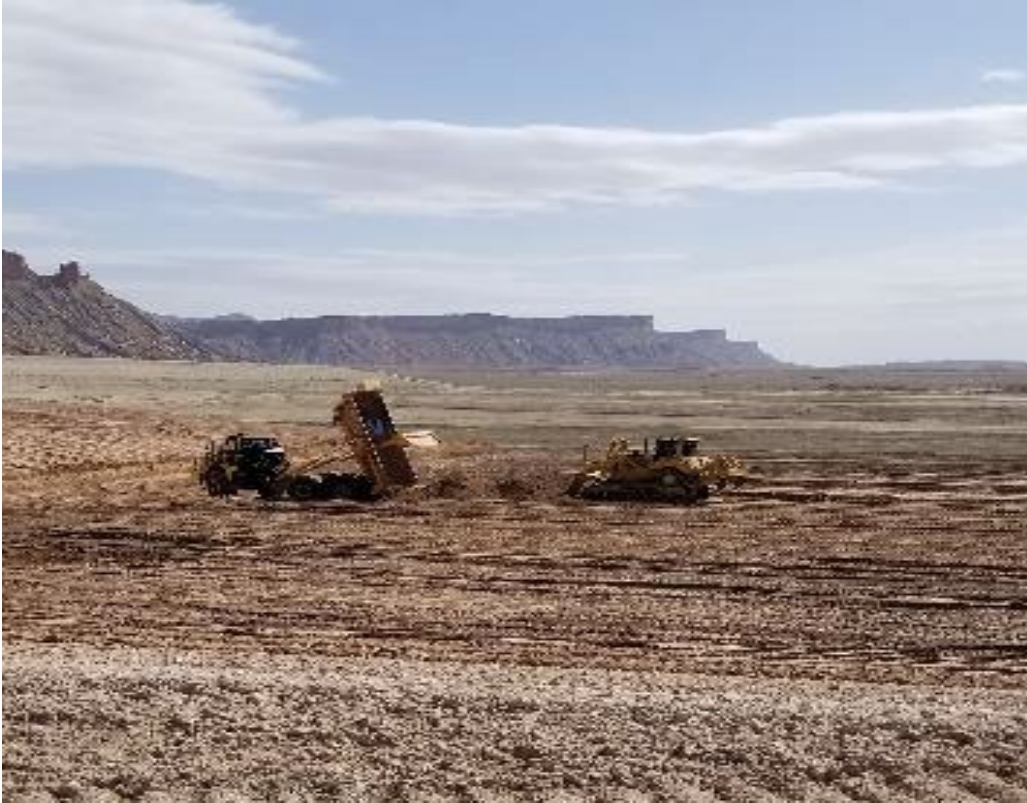
Photo 45. Dozer Pushing Load from Artic Truck May 2022
