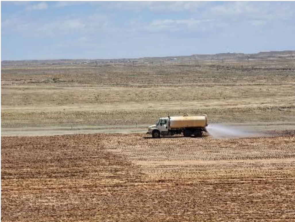
Photo 38. Moisture Conditioning RRM April 2022
