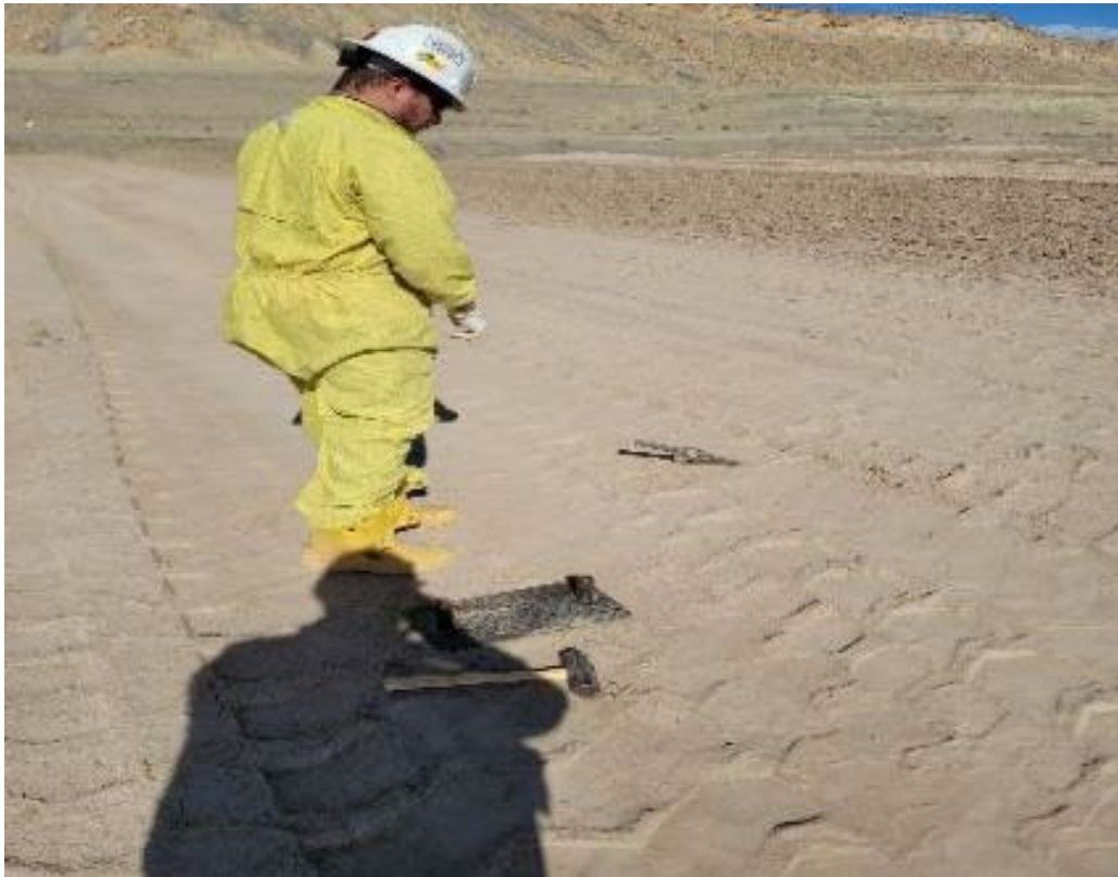
Photo 12. Moisture Density Testing November 2021
