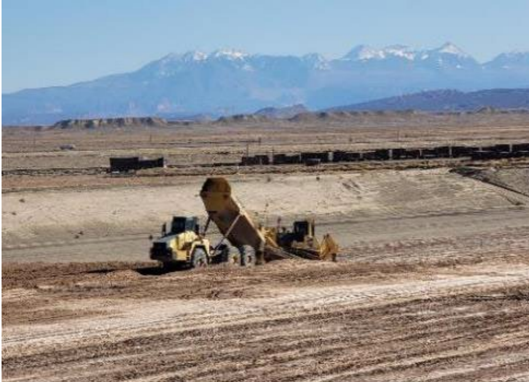
Photo 7. Placing RRM November 2021
