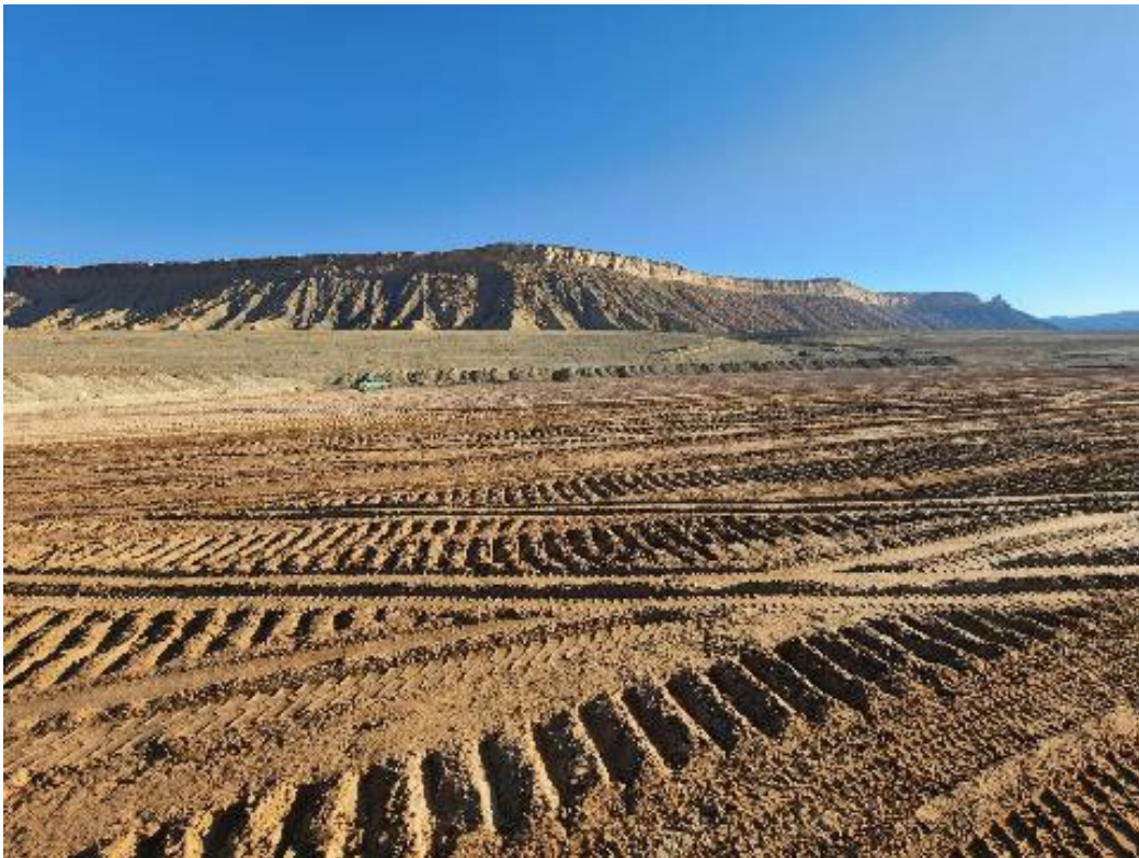
Photo 66. Graded TOW August 2022
