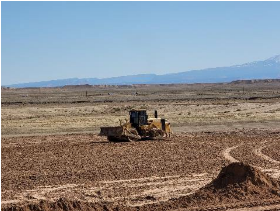
Photo 2. Compacting RRM October 2021
