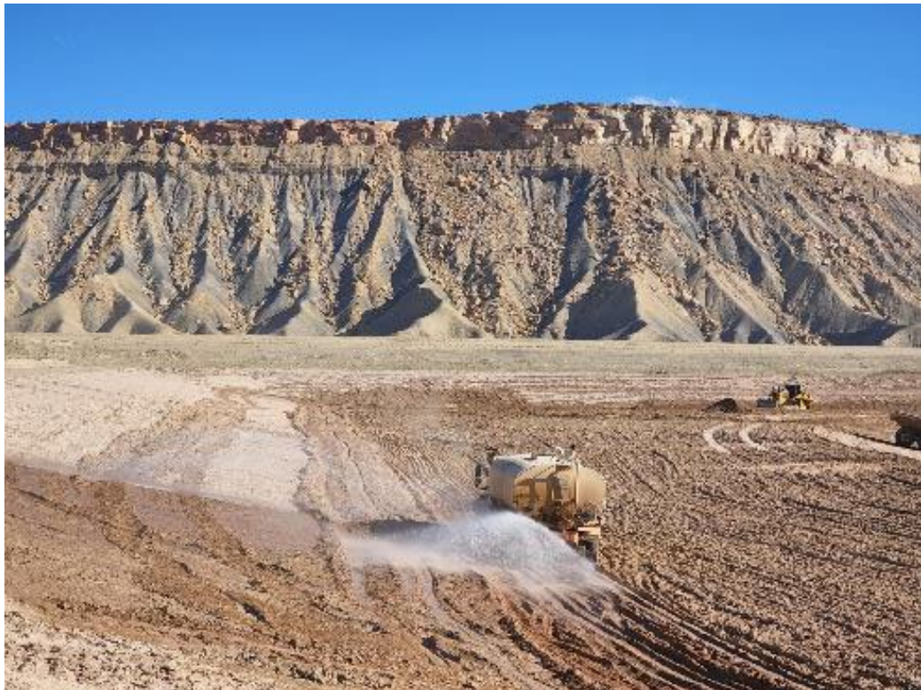
Photo 72. Moisture Conditioning Lifts September 2022
