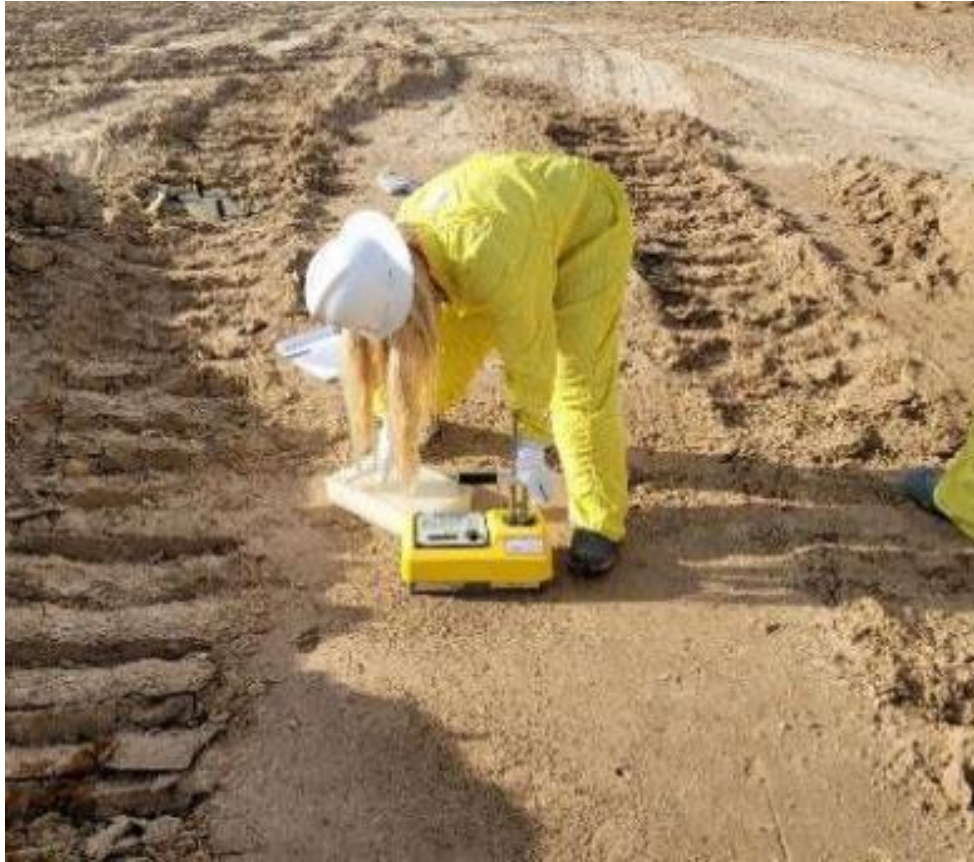
Photo 39. Troxler Testing for Compaction April 2022
