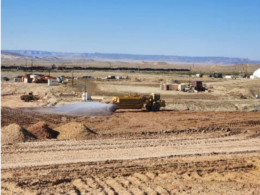
Photo 52 . Moisture Conditioning and Dust Suppression June 2022
