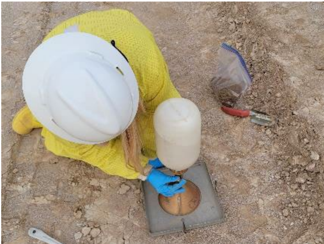
Photo 14. Sand Cone Compaction Testing December 2021
