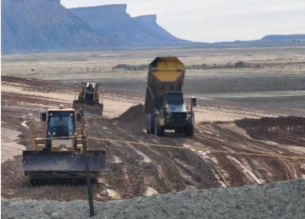
Photo 51. Placing RRM Lift June 2022
