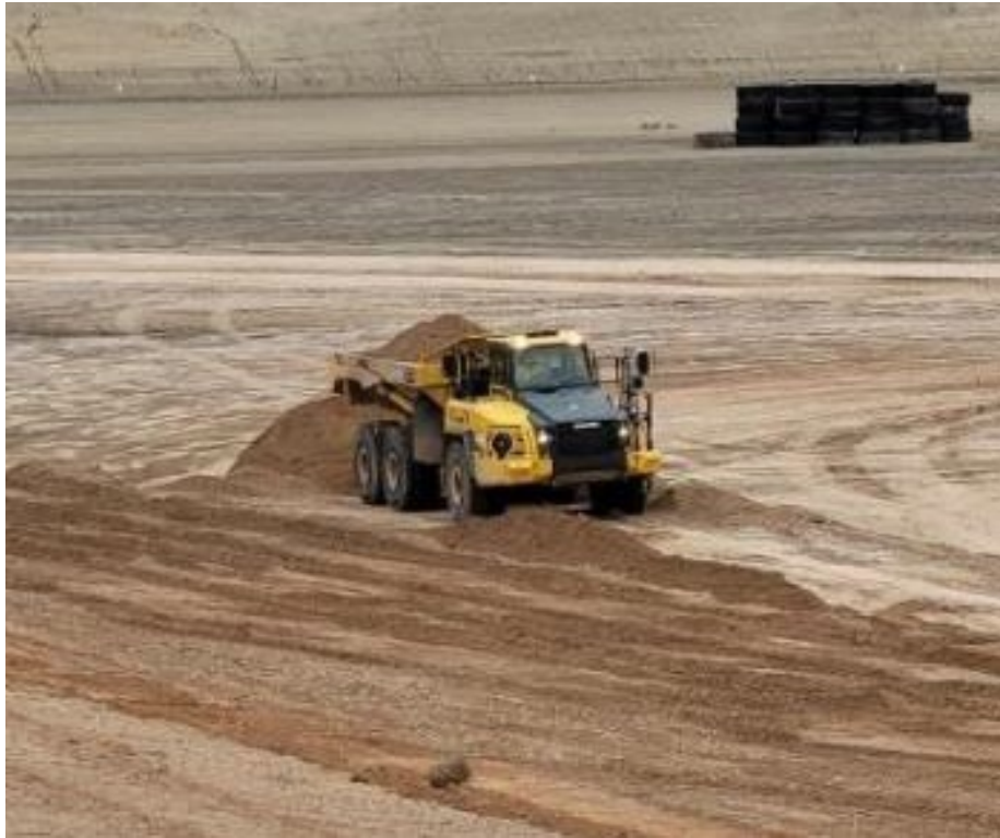
Photo 17. RRM Ready to be Placed December 2021
