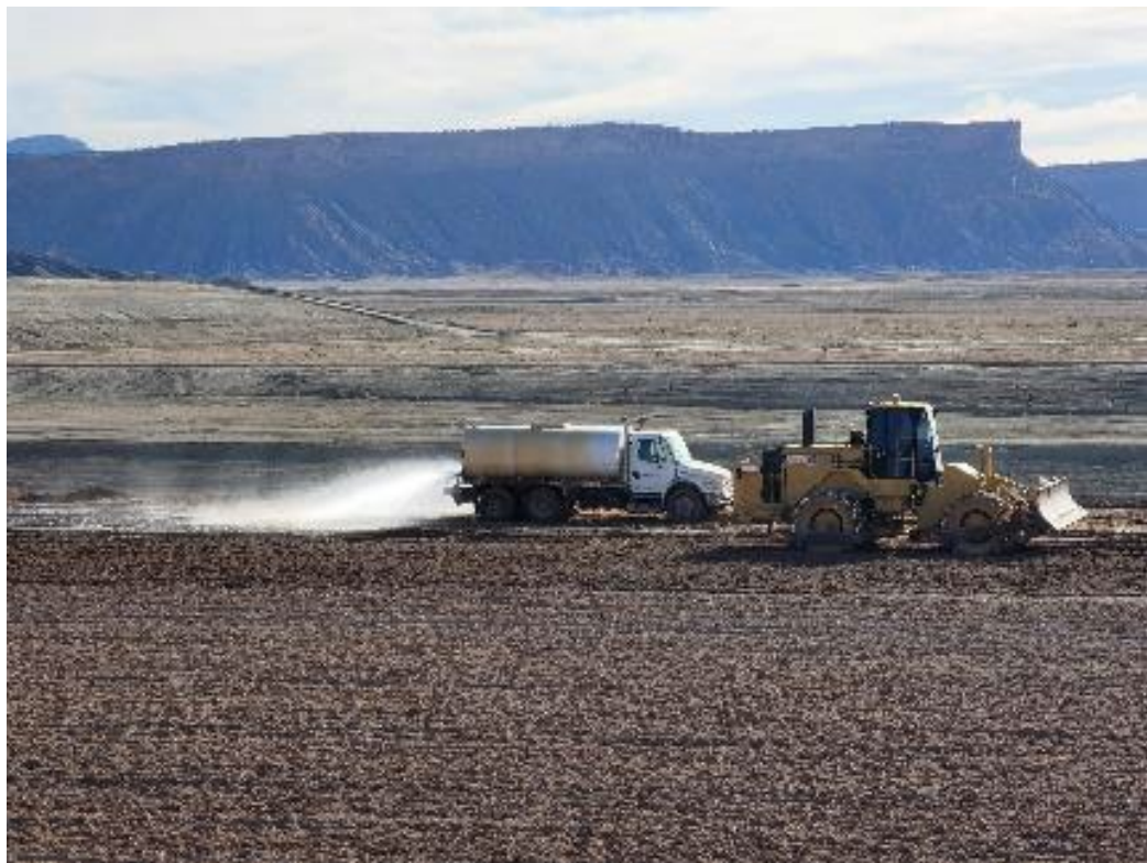
Photo 44. Moisture Conditioning and Compacting RRM Lift May 2022
