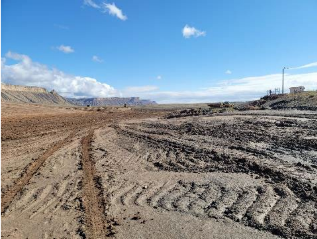
Photo 5. Cell Floor by Water Loadout October 2021
