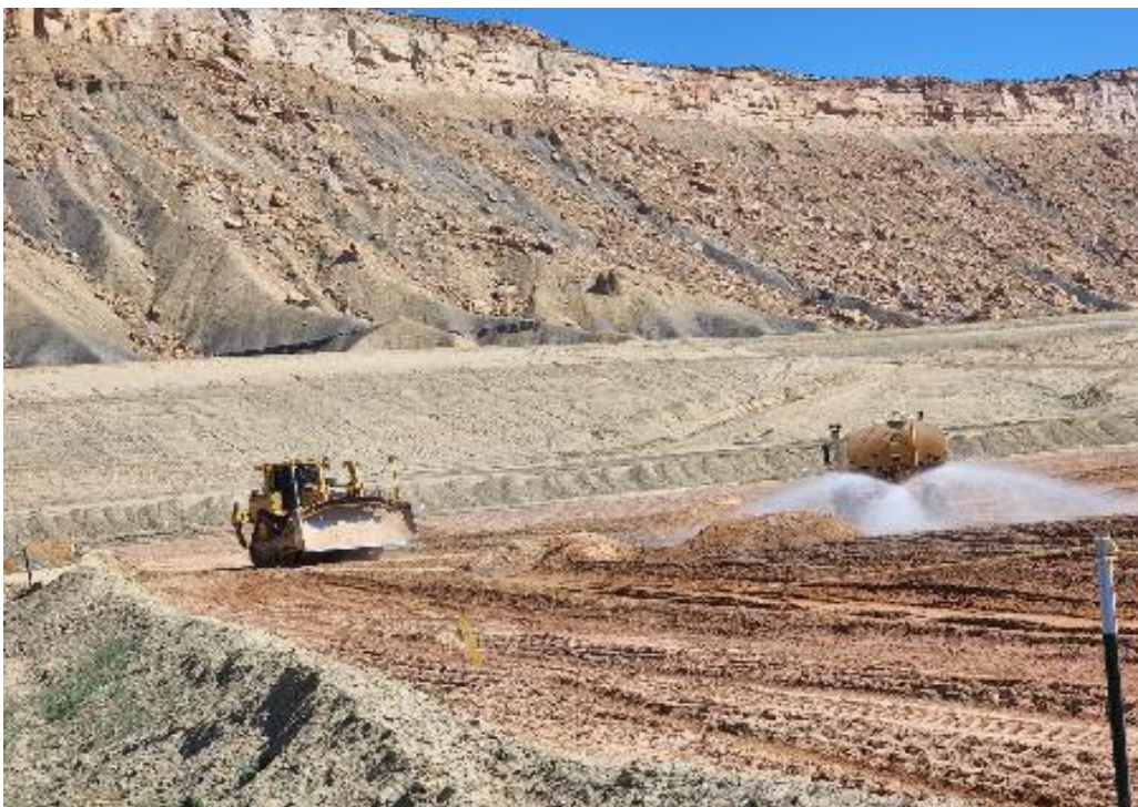
Photo 64. Grading TOW August 2022
