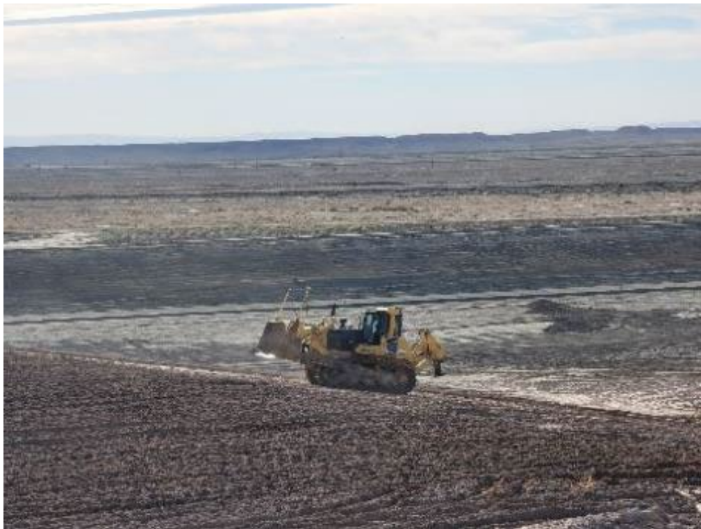
Photo 48. Dozer Climbing up to Lift May 2022
