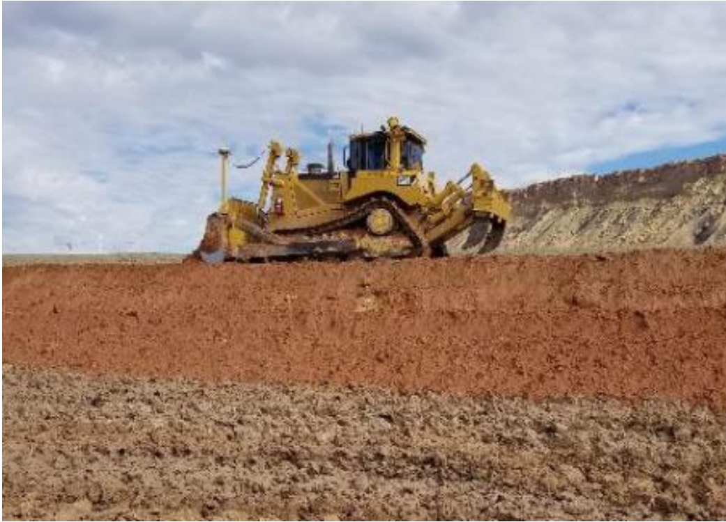
Photo 59. Dozer Cleaning up Stockpile Looking East July 2022
