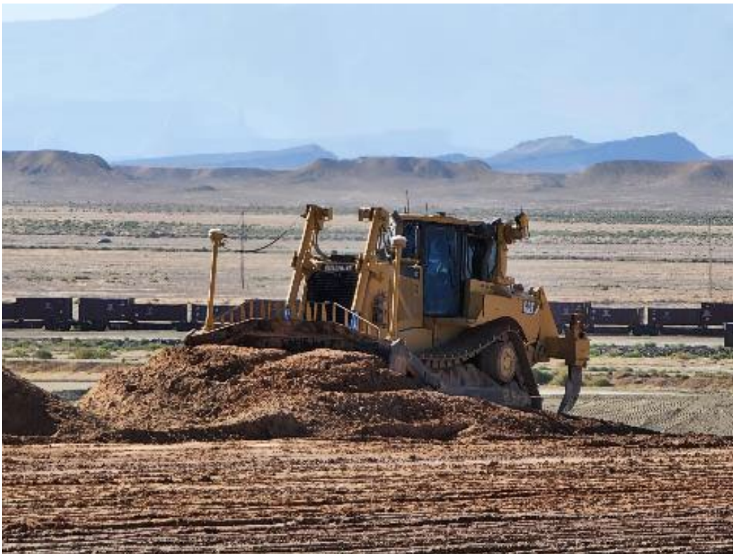
Photo 54. Pushing on RRM Lift June 2022
