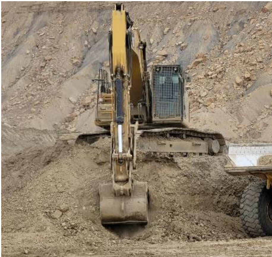
Photo 18. Spoils Stockpile Hauling to North side of Cell December 2021
