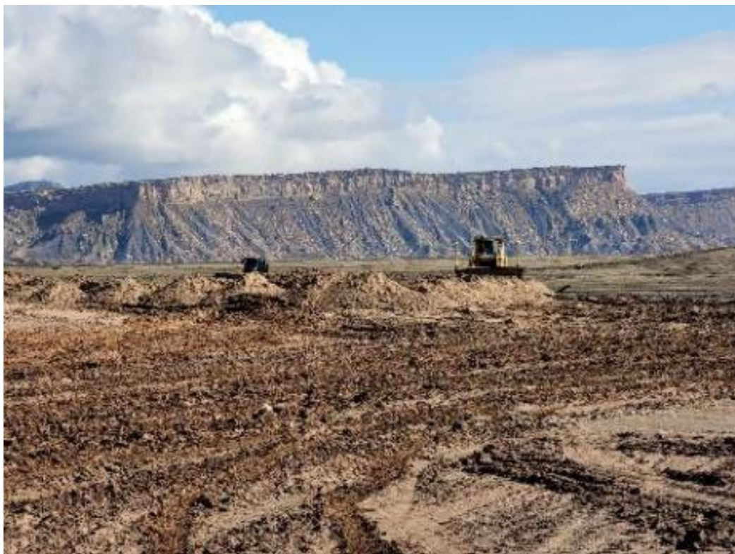
Photo 4. Stock Piling RRM October 2021
