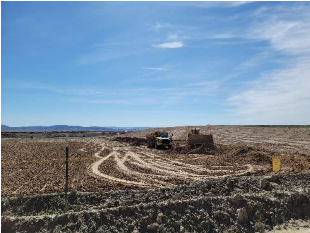
Photo 6. Pushing RRM on RRM Lift October 2021
