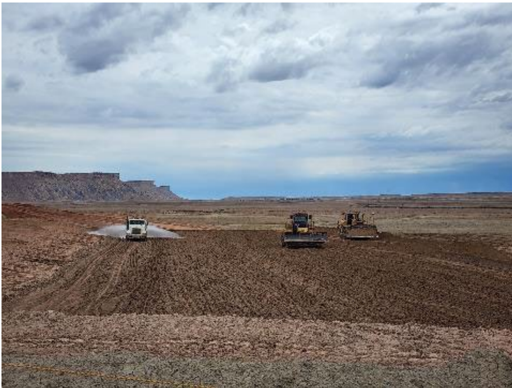
Photo 50. Pushing and Compacting RRM Lift June 2022
