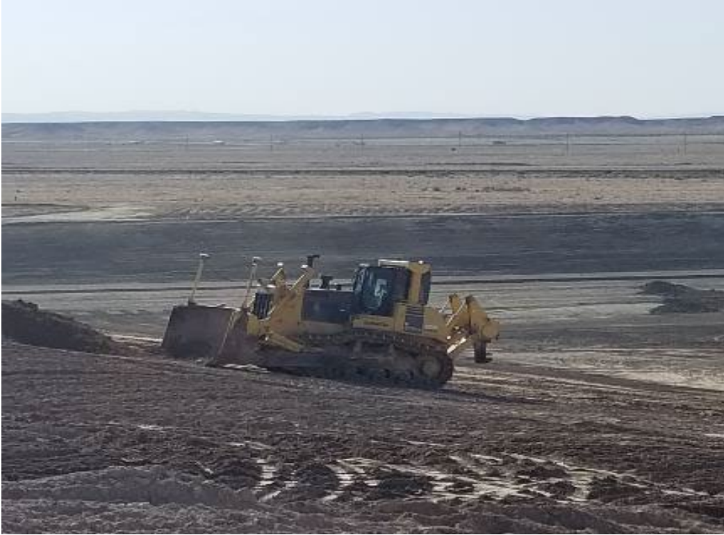
Photo 43. Dozer Waiting for RRM May 2022
