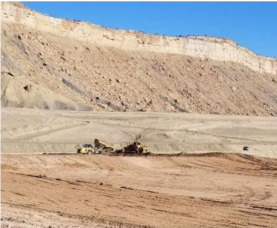
Photo 20. Placing RRM in Top Seven Feet January 2022
