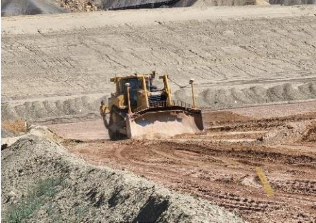
Photo 65. Grading TOW August 2022
