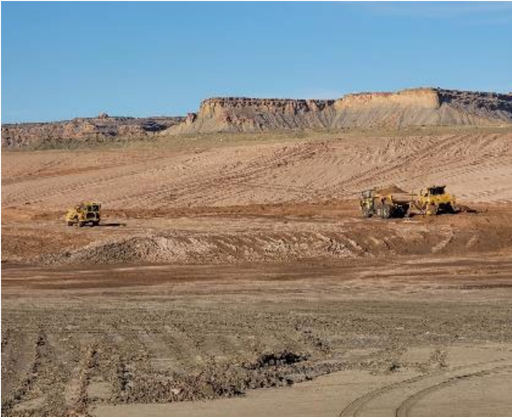
Photo 27. Placing RRM February 2022
