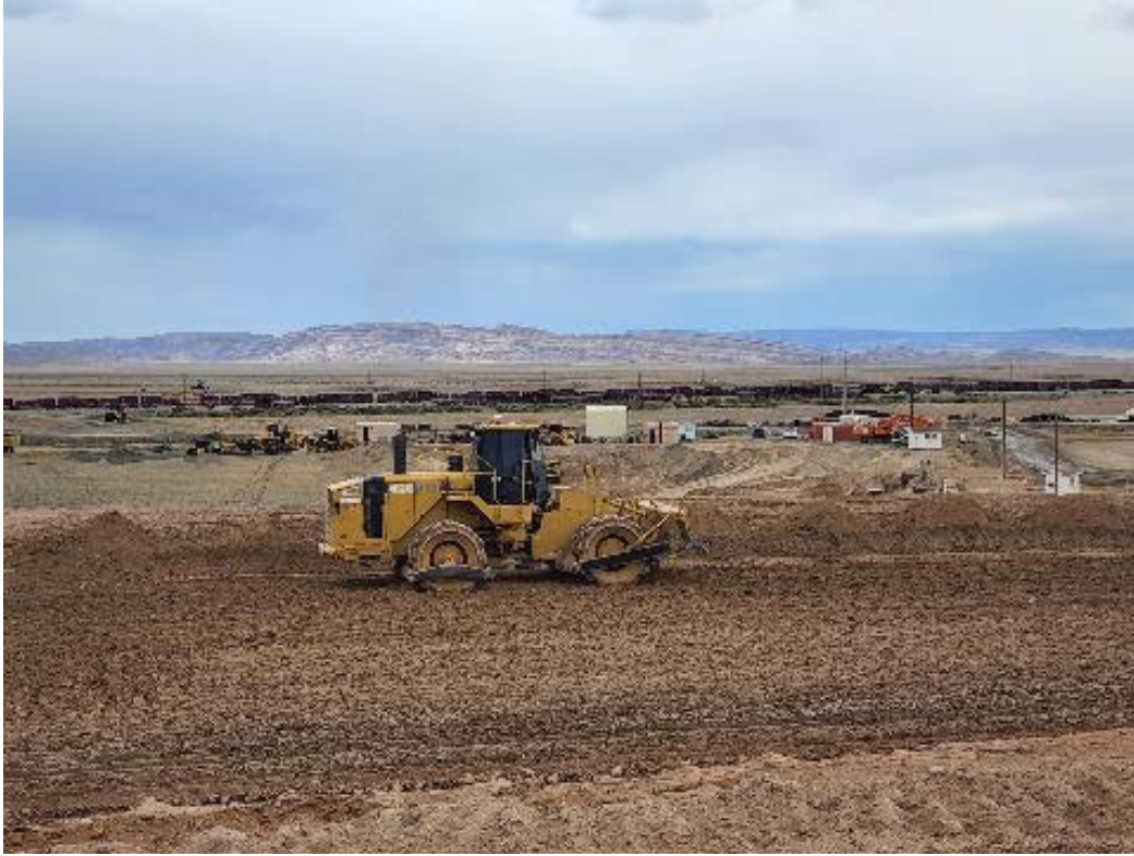
Photo 53 Compacting Lift June 2022
