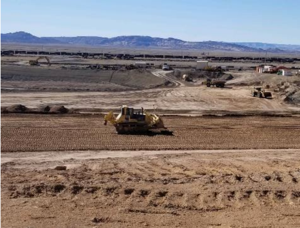
Photo 35. Working RRM Lift March 2022
