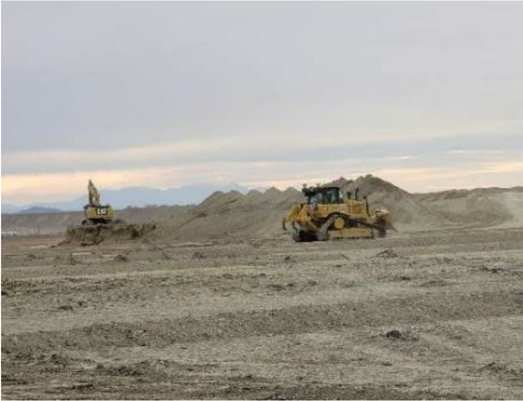
Photo 75. Interim Cover Looking Southwest November 2021
