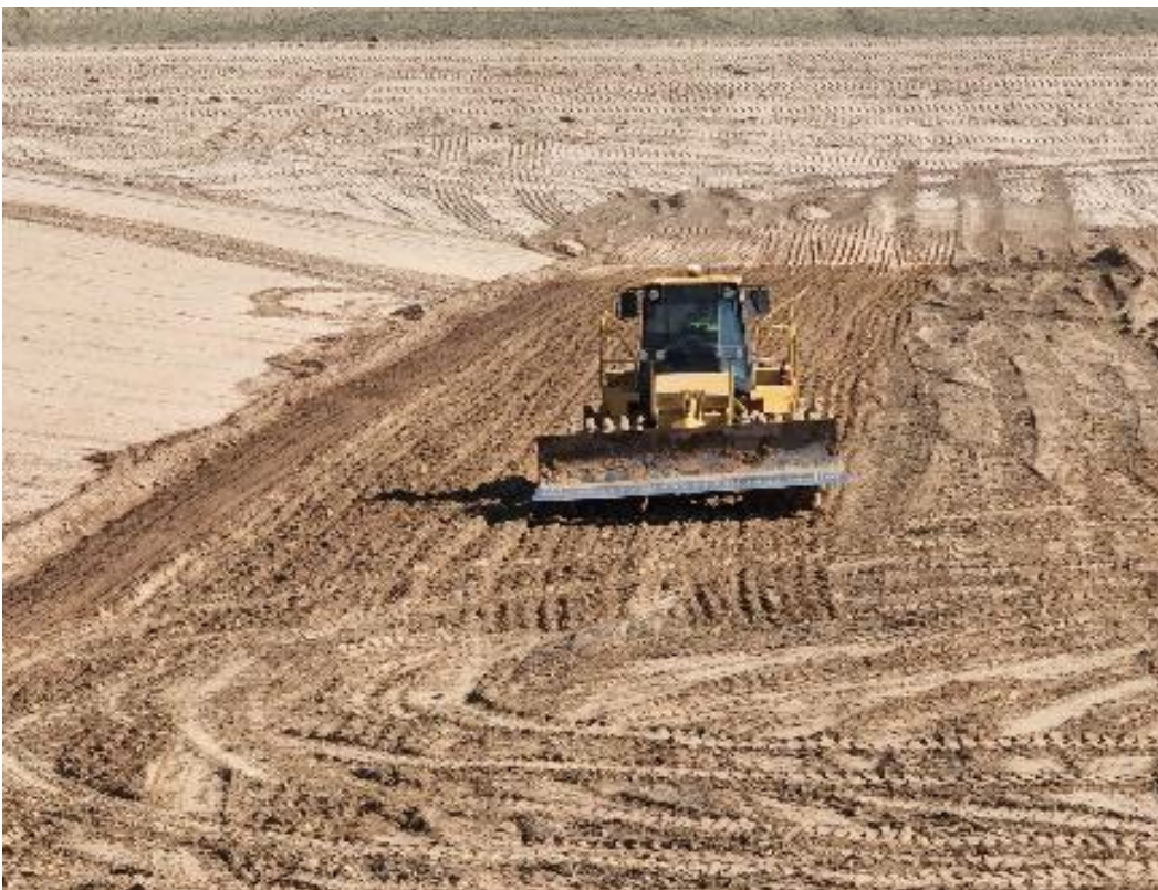
Photo 56. Compacting Looking East July 2022
