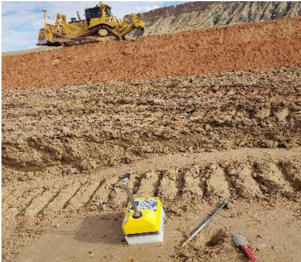
Photo 60. Cleaning up Stockpile July 2022
