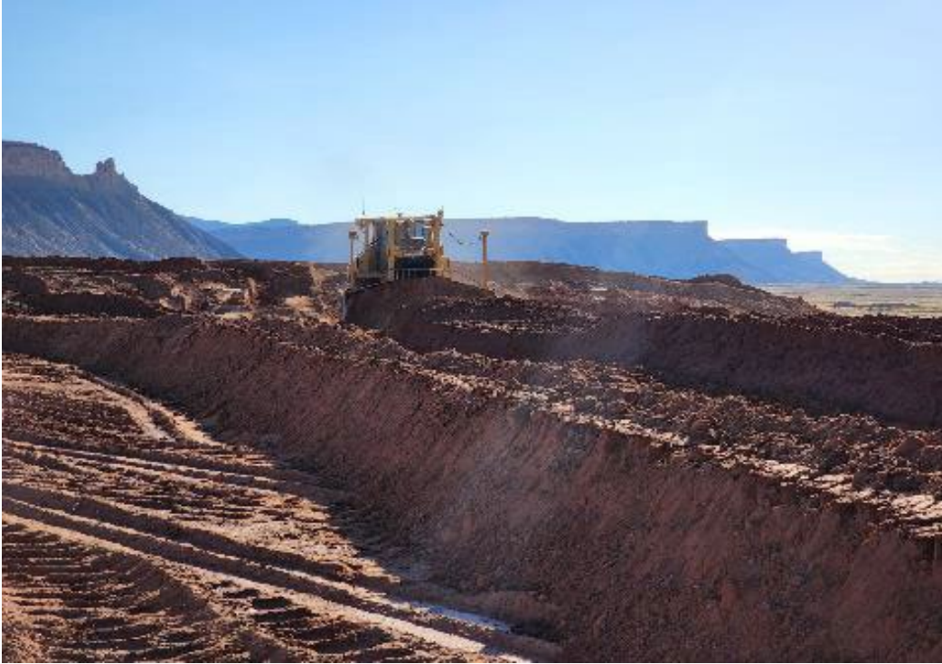
Photo 57. Pushing Stockpile onto RRM Lift July 2022
