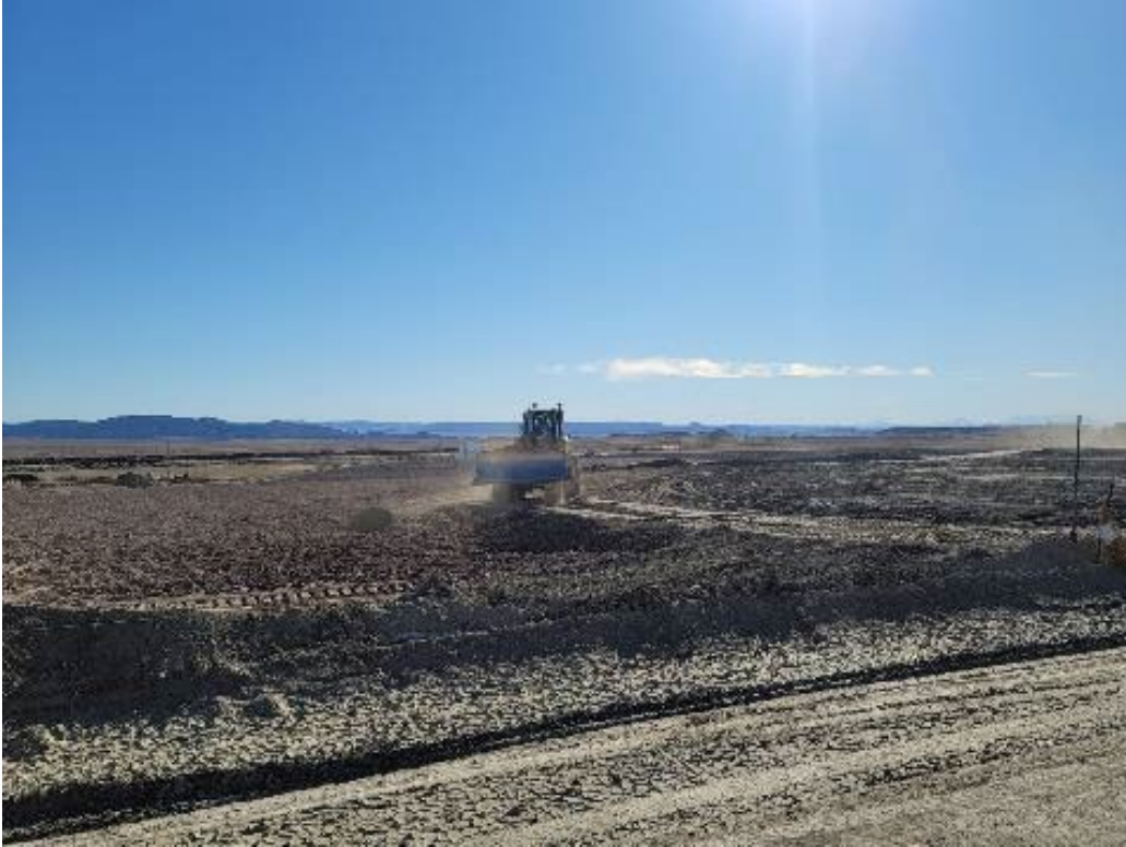
Photo 73. Pushing Interim Lift Looking Southwest November 2021
