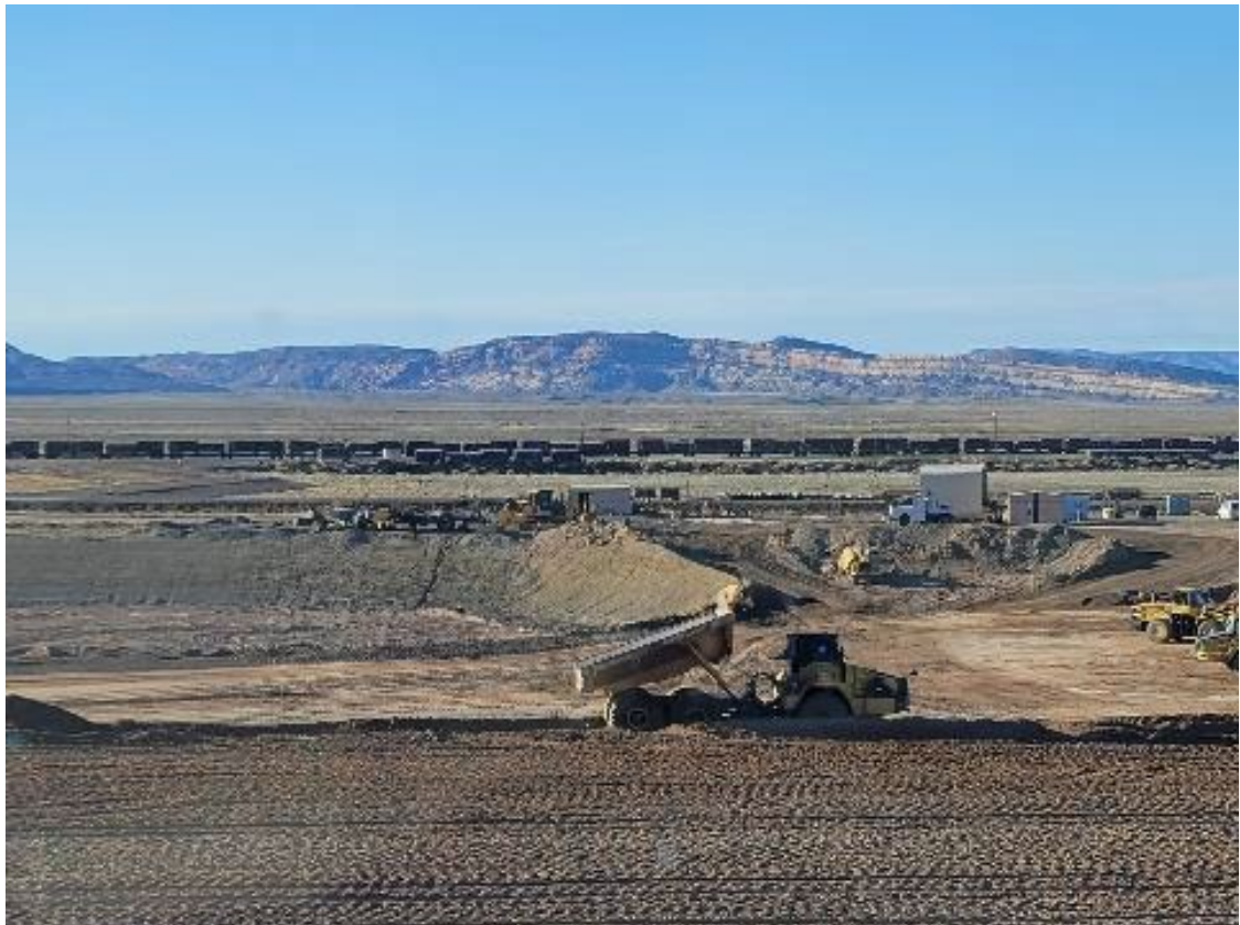
Photo 42. Dumping RRM on Lift April 2022
