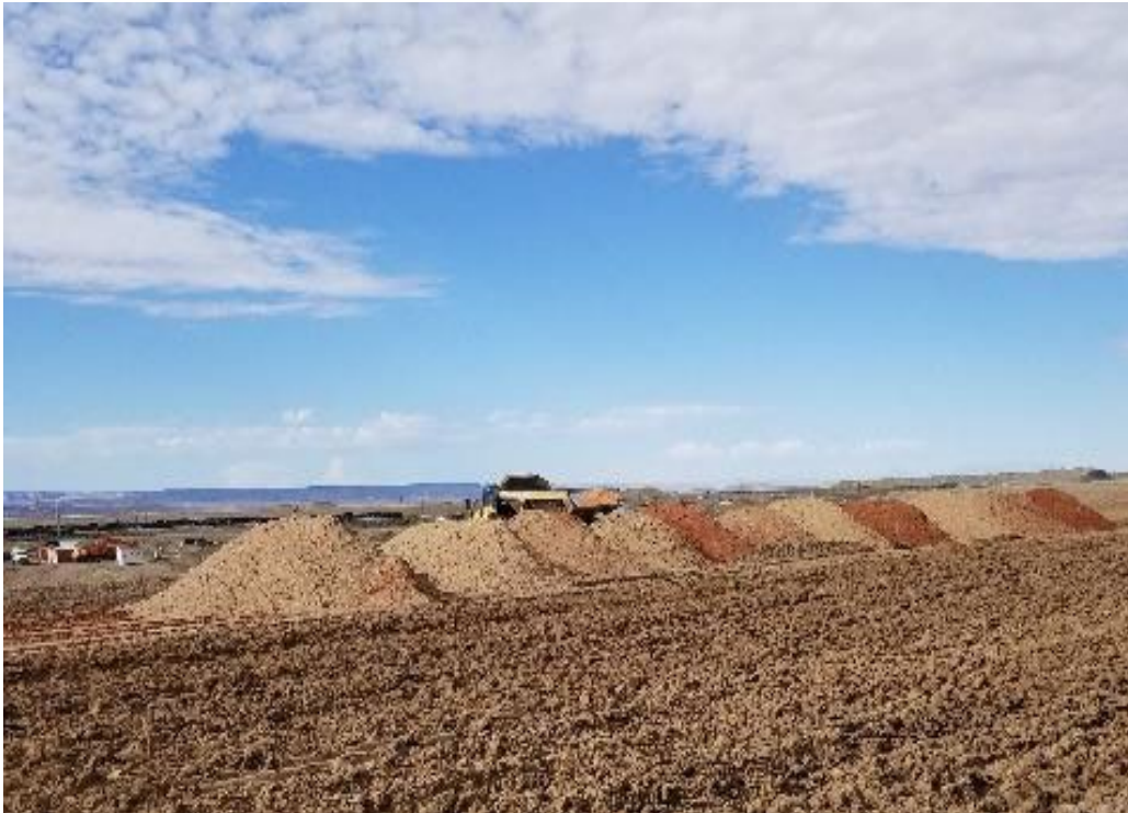
Photo 58. Dumping RRM on Lift July 2022
