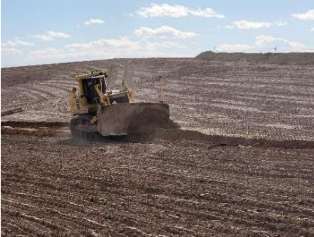
Photo 3. Dozer Keying in RRM Lift October 2021
