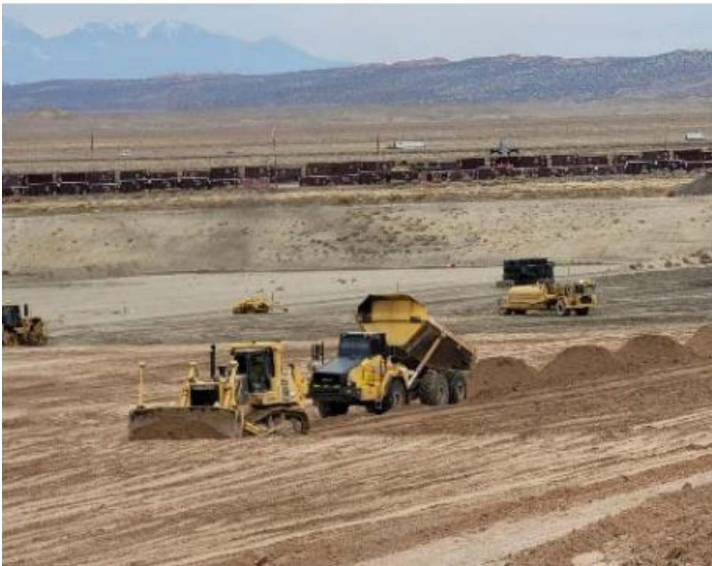
Photo 8. Placing and Pushing RRM November 2021
