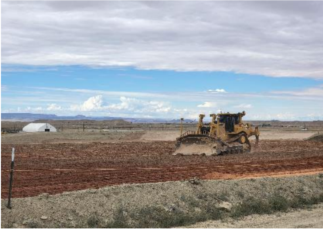
Photo 61. Grading Top of Waste August 2022
