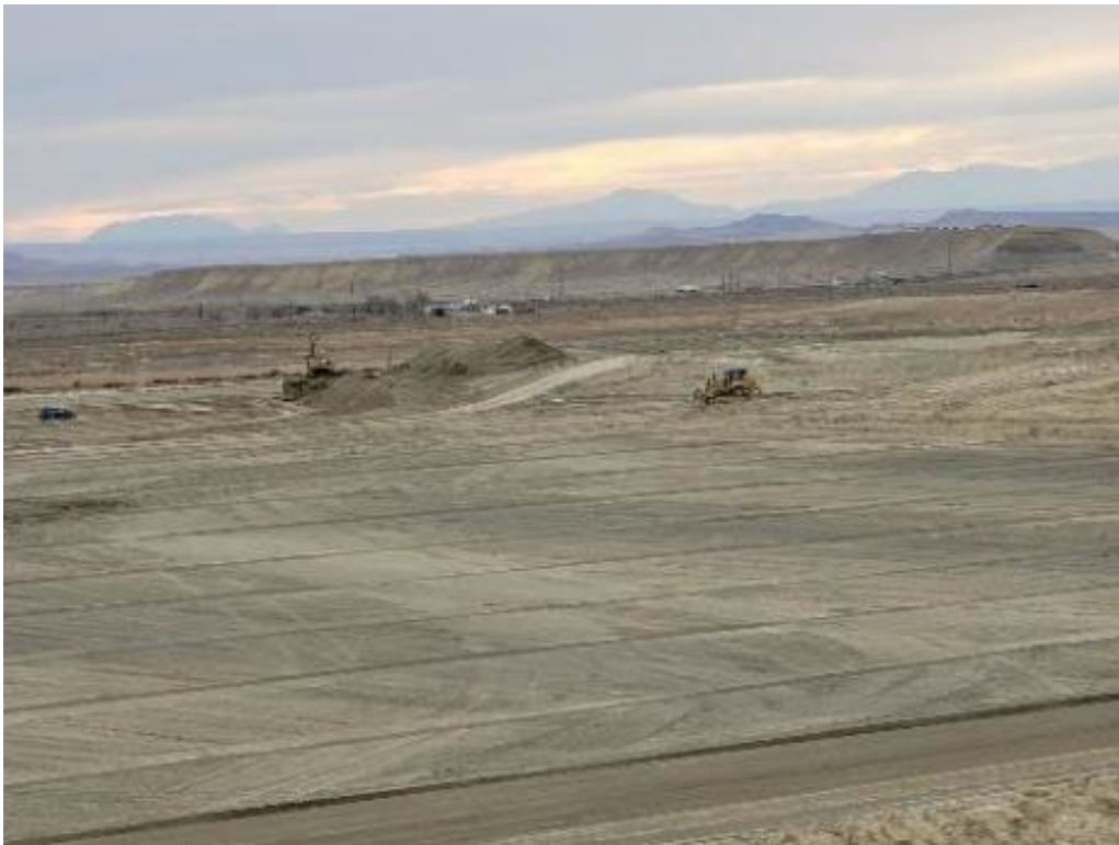
Photo 76. Interim Cover Looking Southwest November 2021
