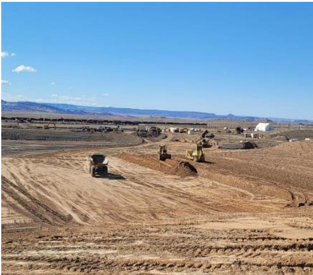
Photo 32. Disposal Cell Operations March 2022
