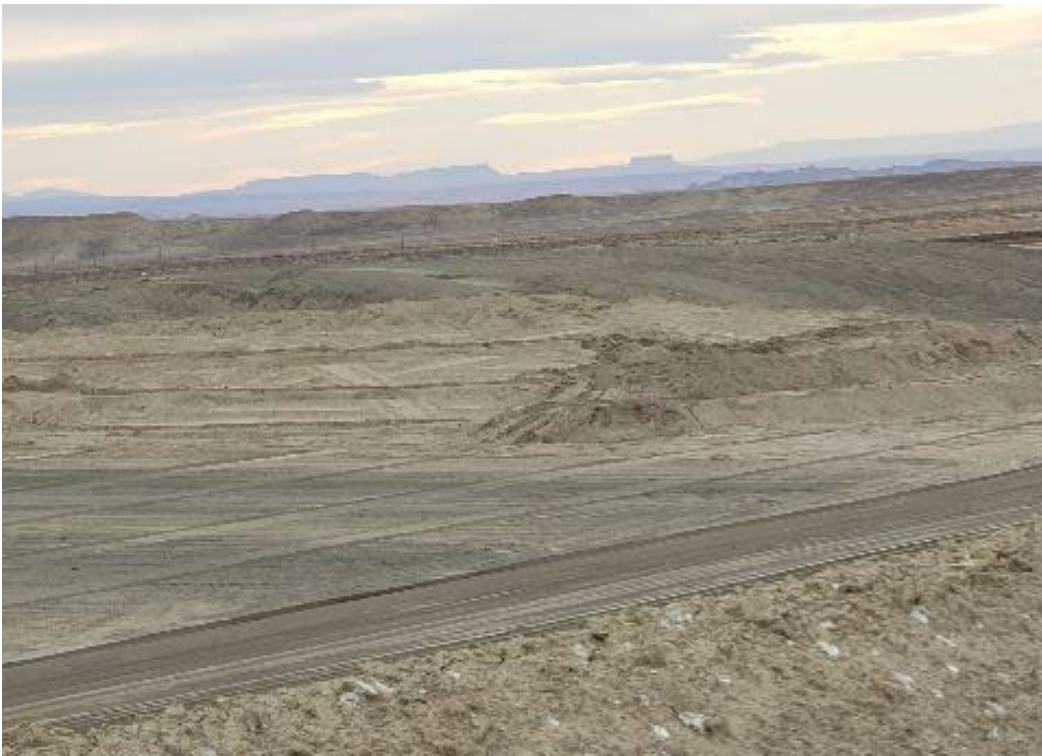
Photo 74. Spoils Pile Material for Interim Lift November 2021
