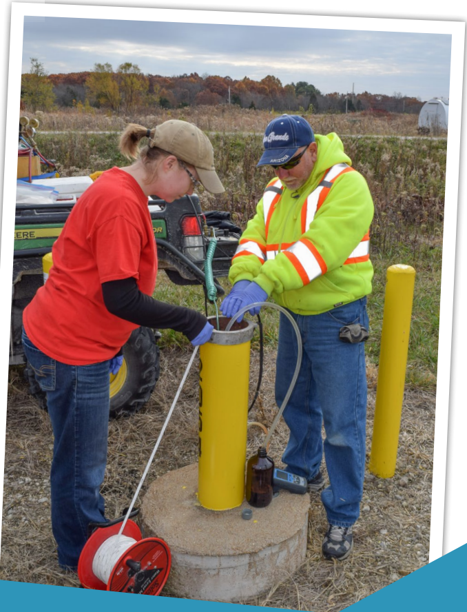
Groundwater monitoring at St. Charles County, Missouri. ▶
