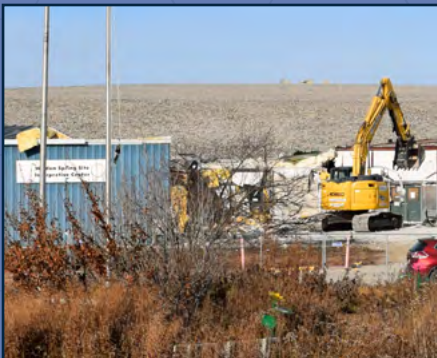
USACE begins demolishing the former Weldon Spring Site Interpretive Center.
