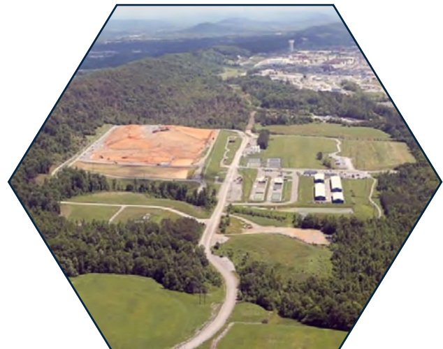
EM Waste Management Facility at Oak Ridge.
