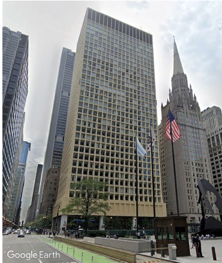
Figure 1. Image of George W. Dunne Building in downtown Chicago, IL.
