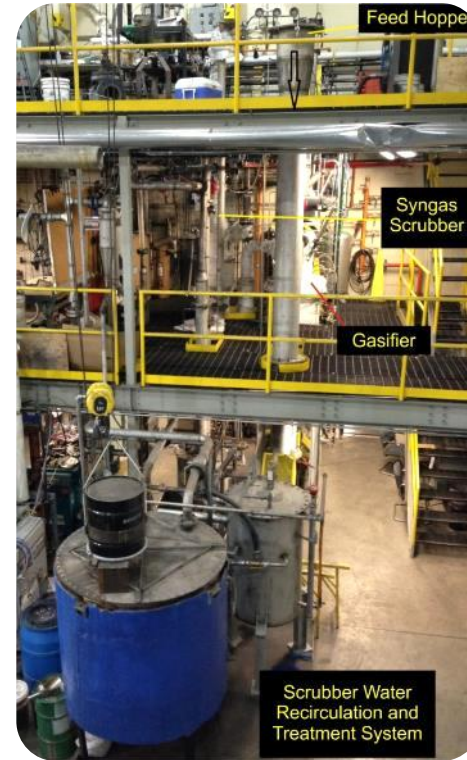
Downdraft Fixed-Bed Gasification (DFB)
