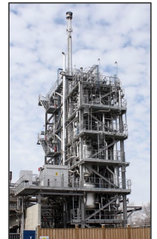
Gasification/DME pilot plant (ltu.se)
