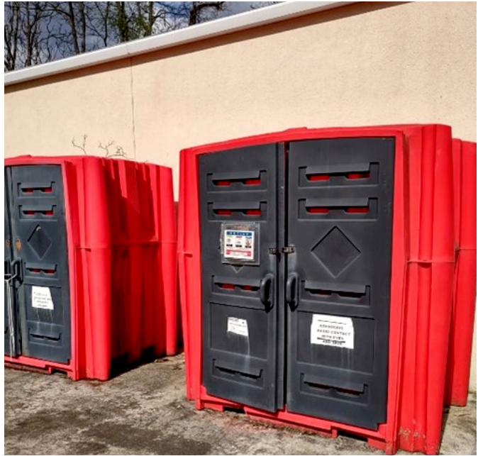
FIGURE 9 | Acid and base dispensing sheds for wastewater discharge pH treatment at NETL
