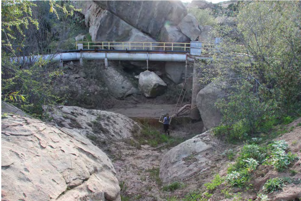
R2-A Photo 1. View of west end of the impoundment showing shallow water level on February 25, 2010, maintained at this low level by pumping.
