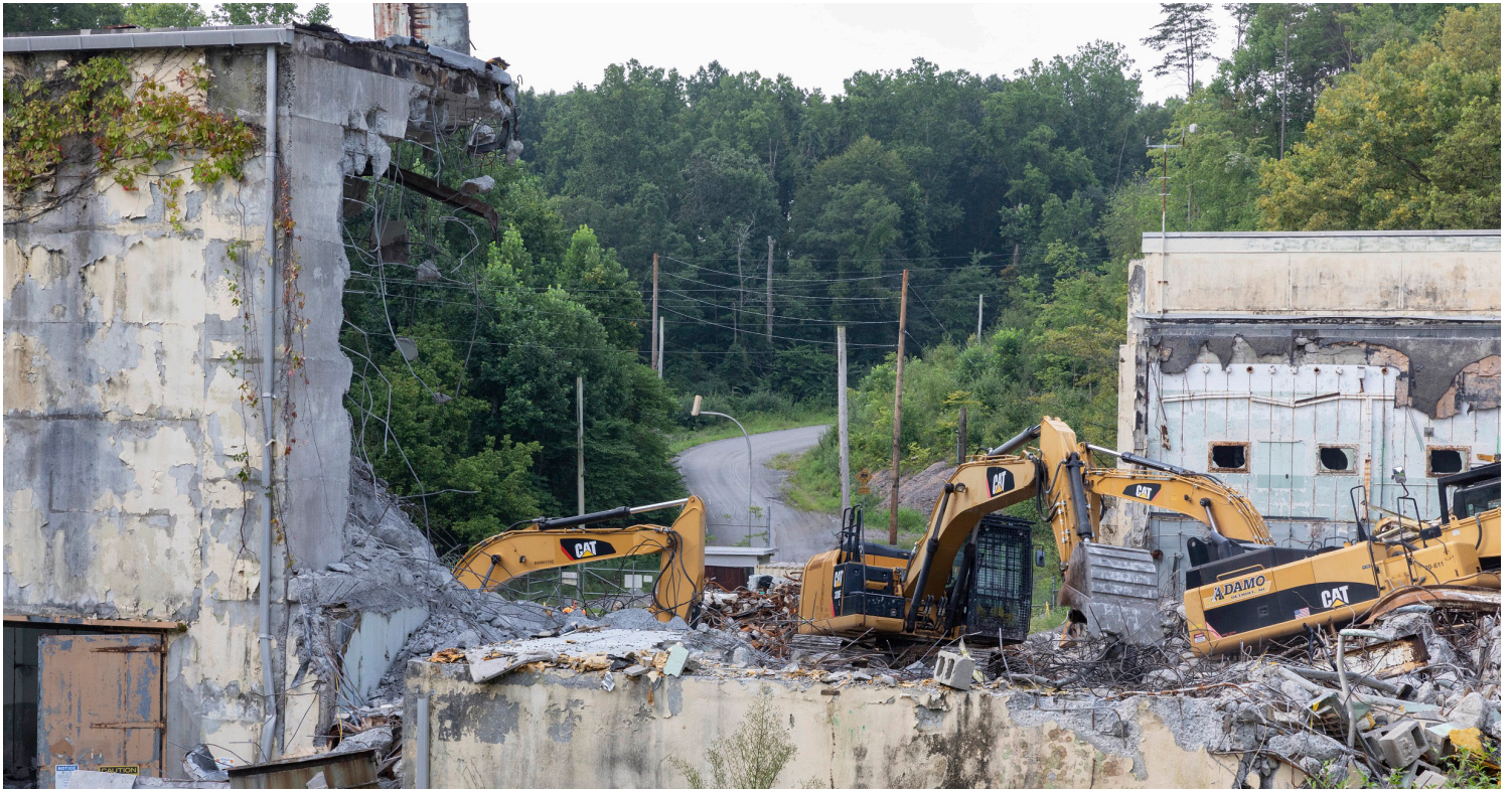
A view of crews demolishing the Criticality Experiment Laboratory at Y-12.
