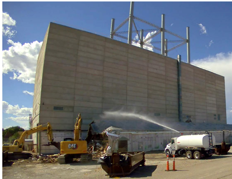
Crews demolish buildings B608/625 at the NRF.
