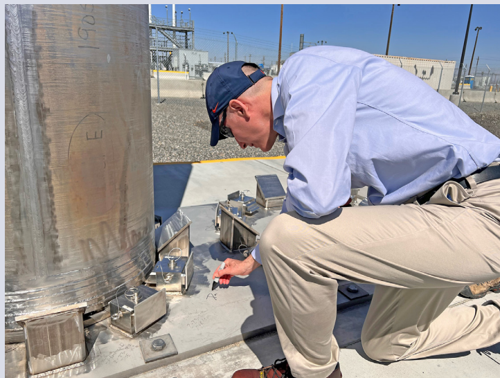
Deputy Energy Secretary David Turk signs his name on concrete next to a shielded container to mark Hanford Site's progress in treating waste from underground tanks with the Tank-Side Cesium Removal System.
