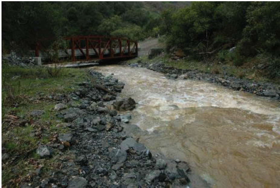
Figure E-9. Flooding Event at Arroyo Mocho
