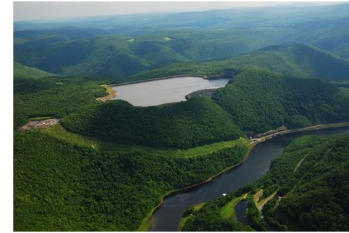
Bear Swamp Pumped Storage Hydro
