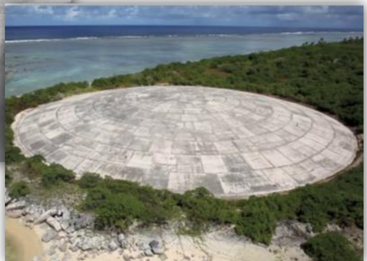
Cactus Crater before (left) and after (right) construction of the Cactus Crater containment structure (i.e., Runit Dome)
