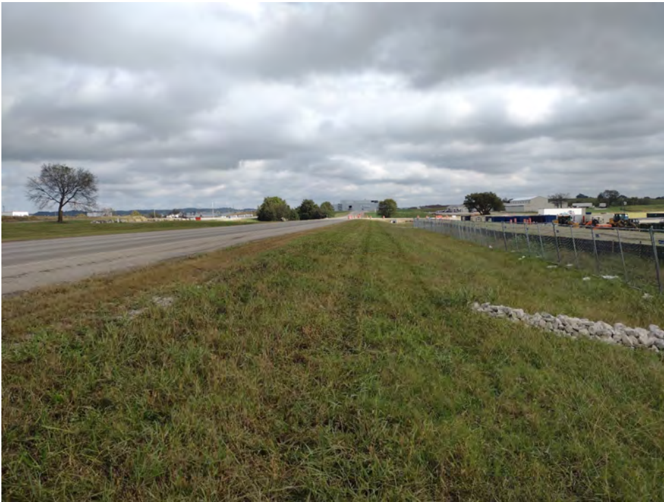
Photograph 1. Overview of Area 3 (southeast edge), facing northeast.
