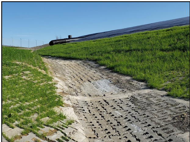
NDA north slope erosion controls
