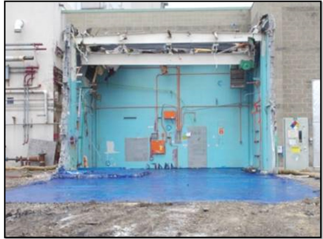
Completed conditions after demolition of the laundry facility
