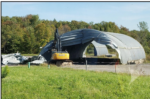
Demolition of the Chemical Process Cell- Waste Storage Area (CPC-WSA)
