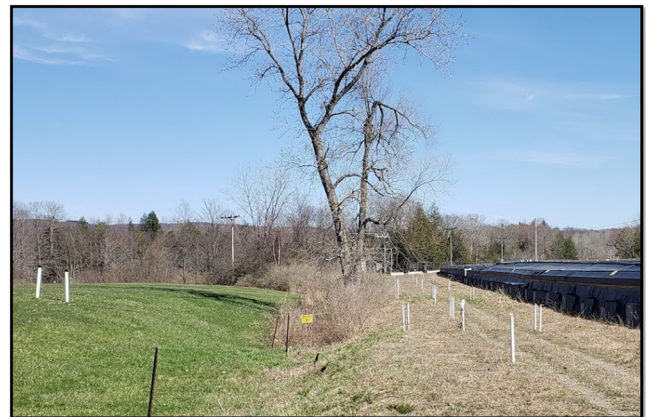
Permeable Treatment Wall (PTW) monitoring wells
