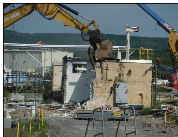
Demolition of the Waste Tank Farm (WTF) shelter
