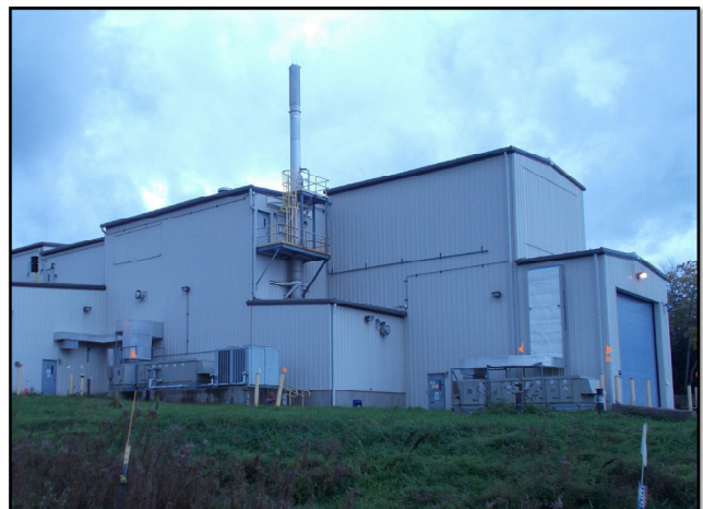
Remote Handled Waste Facility (RHWF) stack
