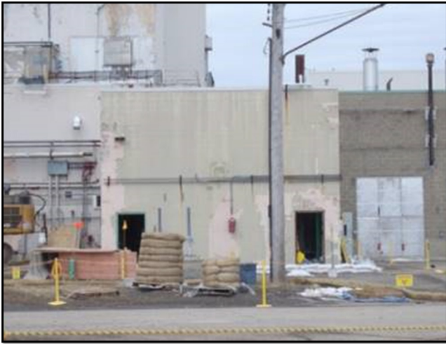
The laundry facility prior to demolition
