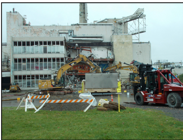
Demolition of the Main Plant Process Building (MPPB) offices in progress
