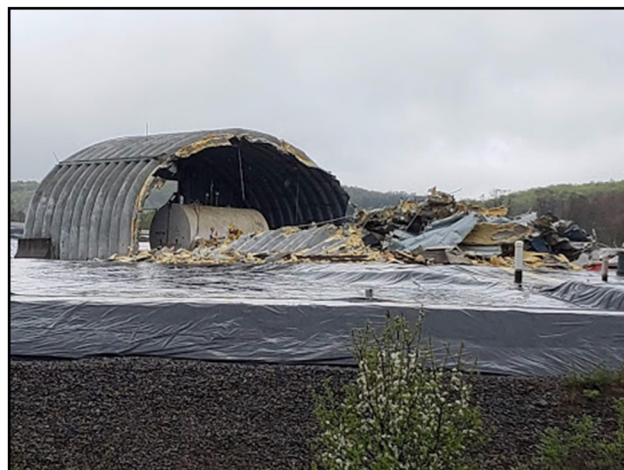
Demolition of the Liquid Pretreatment System (LPS) building
