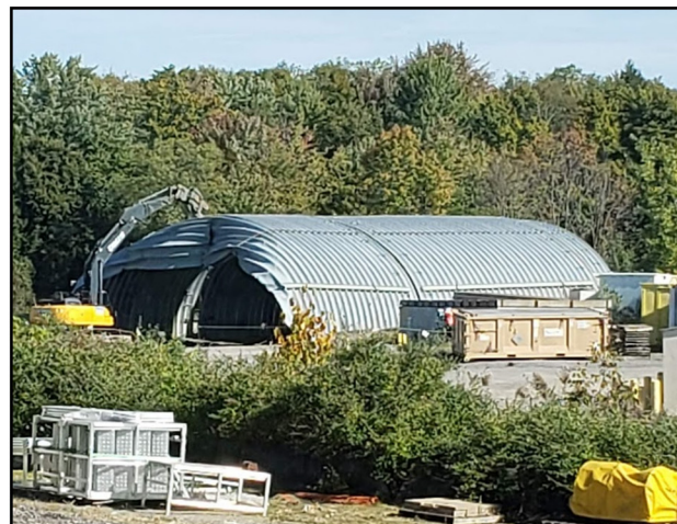
Demolition of the Chemical Process Cell - Waste Storage Area (CPC-WSA)
