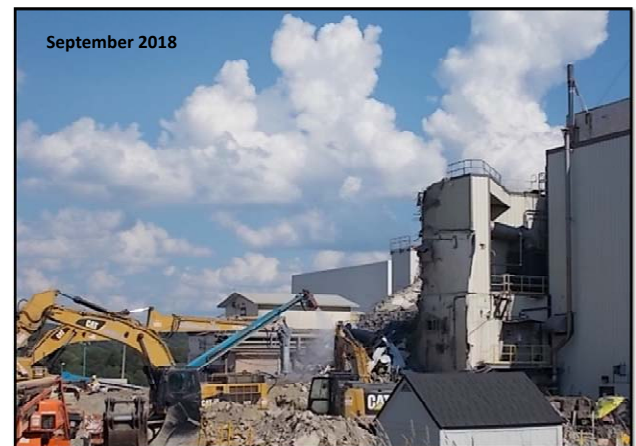
Vitrification Facility (VF) after demolition
