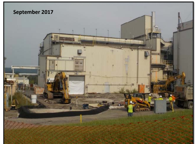
Vitrification Facility (VF) before demolition
