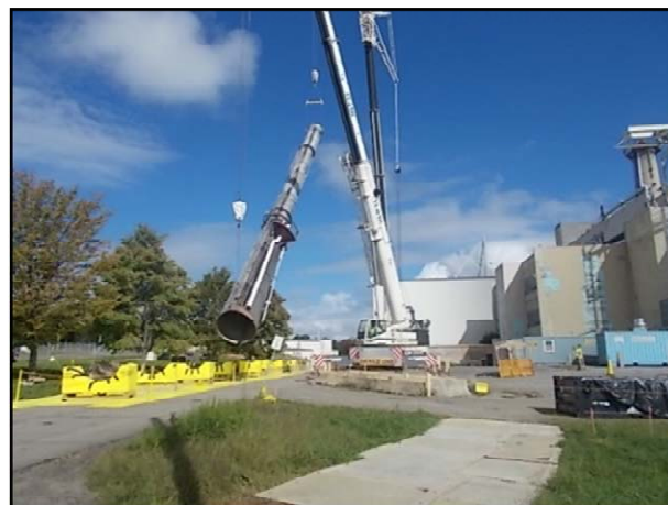
Main Plant Process Building (MPPB) stack being prepared for disposal
