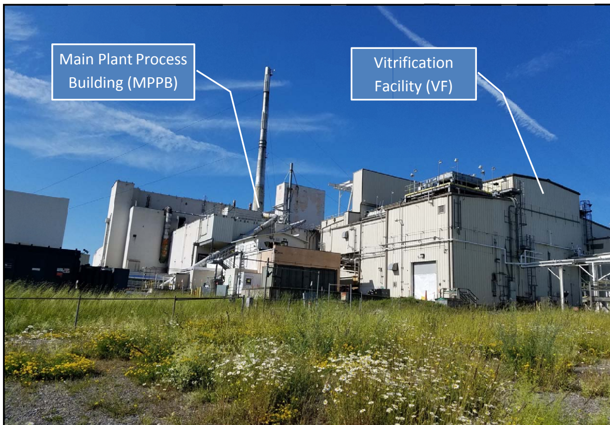
Vitrification Facility (VF) and Main Plant Process Building (MPPB)
