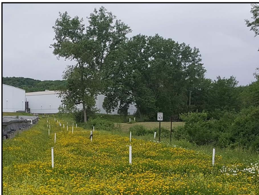
Permeable Treatment Wall (PTW) monitoring wells
