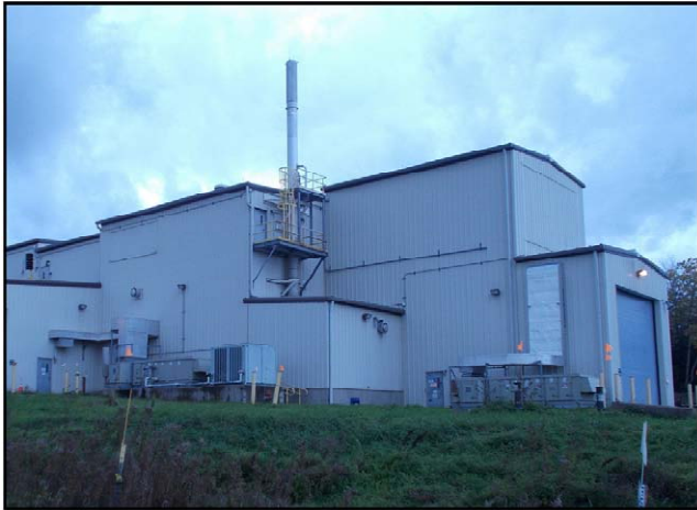
Remote Handled Waste Facility (RHWF) stack
