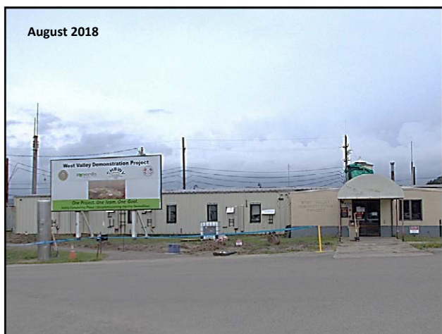
Administration building before demolition
