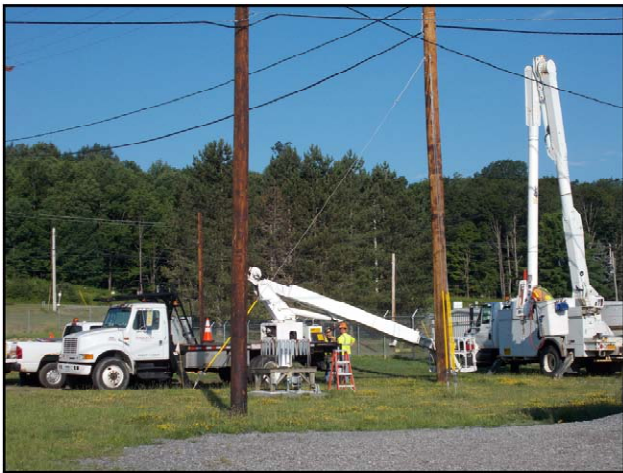
Upgrading electrical infrastructure
