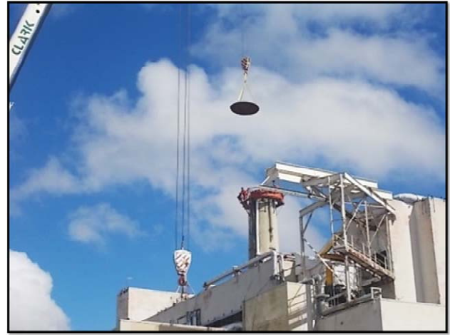
MPPB stack capped after removal above the gunite
