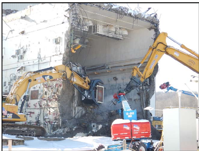
Removal of viewing window during VF demolition
