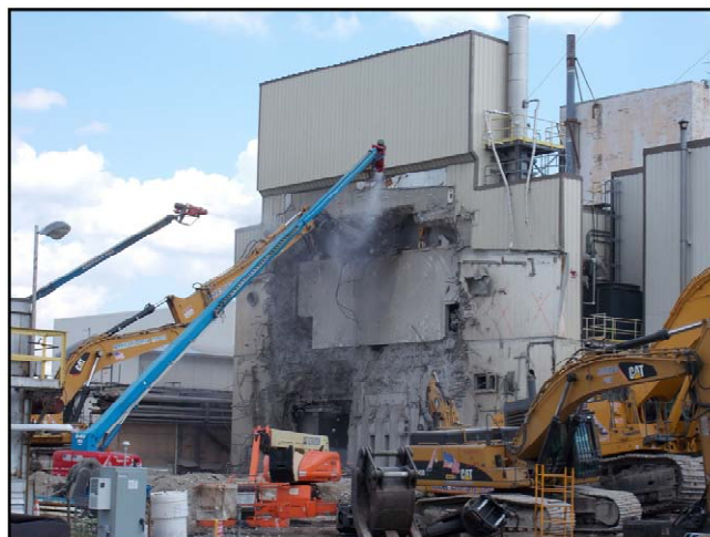
Preparing for removal of the upper VF shield door
