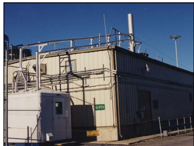
The Tank and Vault Drying System (T&VDS) exhausts through the Supernatant Treatment System (STS) stack
