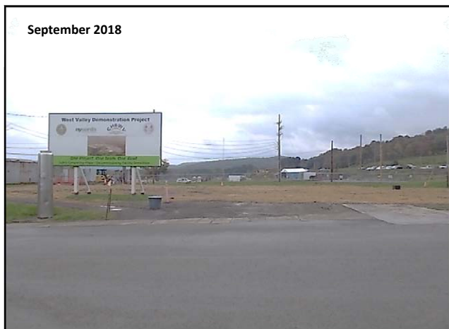
Administration building after demolition
