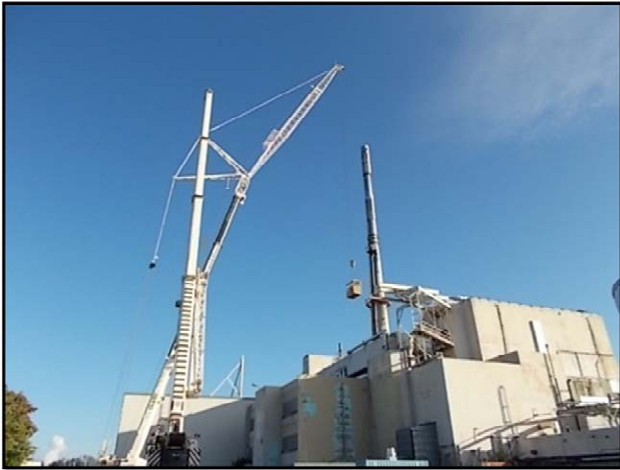
MPPB stack in preparation for removal
