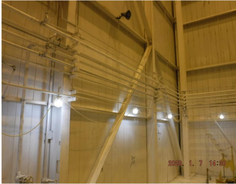
Workers foam piping in FRS to fix contamination
