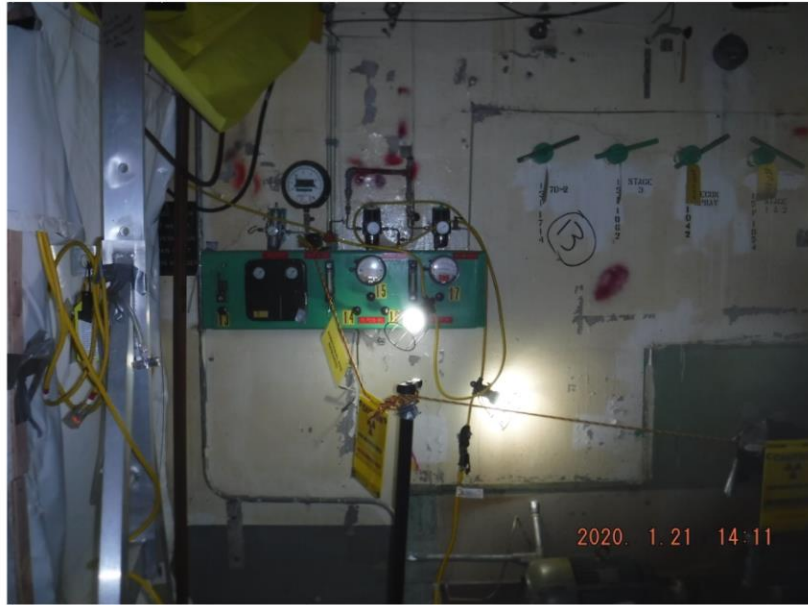
Inside Vent Wash Room
