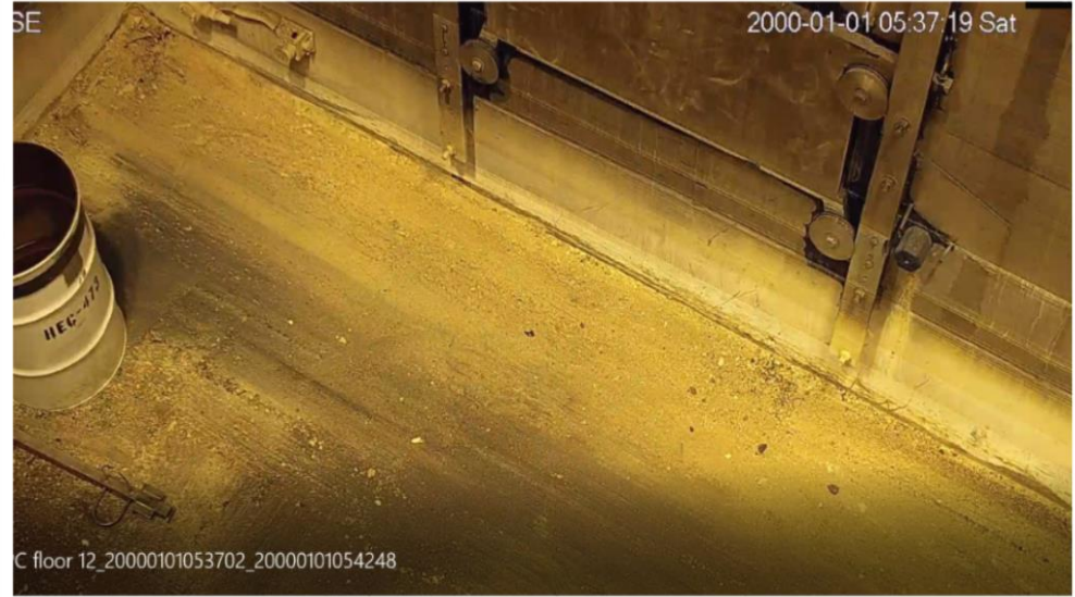
GPC northwest corner cleaning progress
