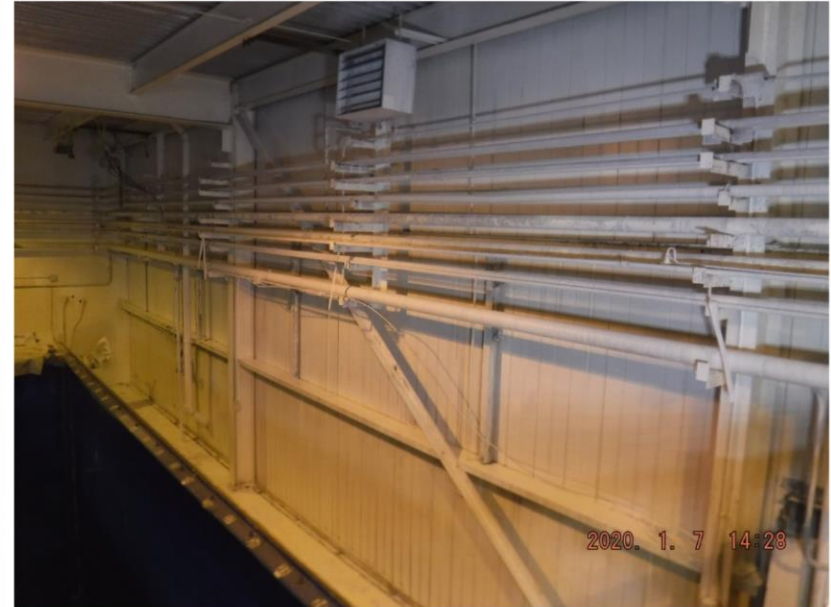
Wooden platform is built to aid in ACM removal
