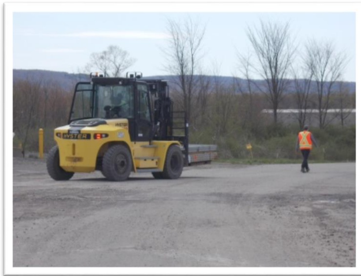
Offloading materials and supplies
