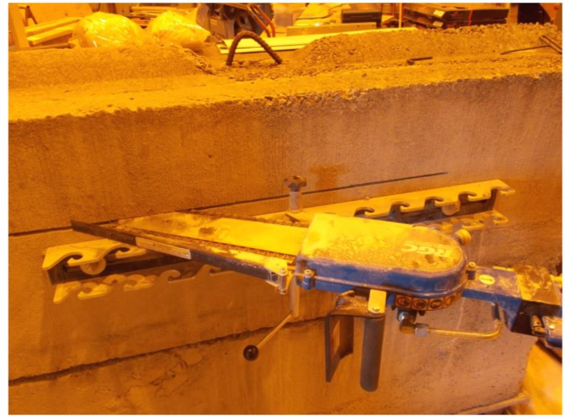
Concrete diamond-cut saw mockup
