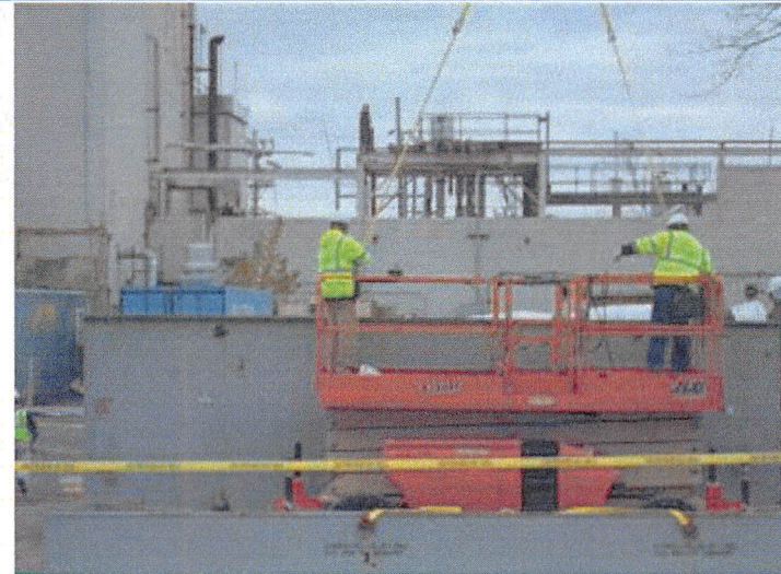
Removing VEC 36-inch duct from MPPB roof
