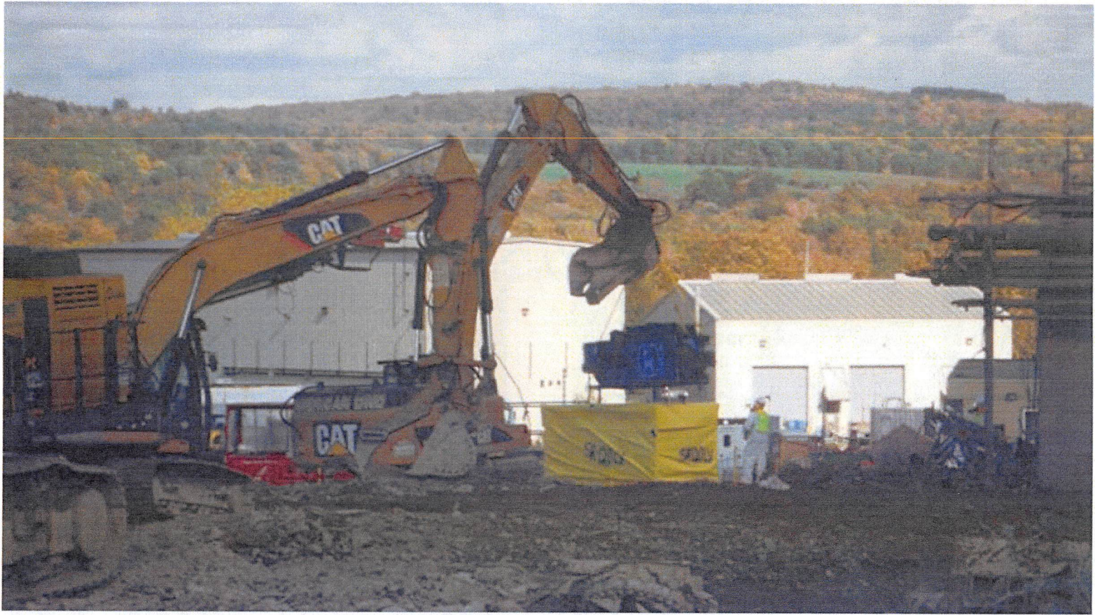
Contact-Size Reduction Facility's dust collector being loaded during demolition
