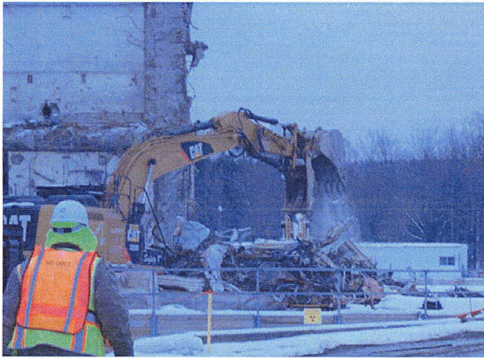
Waste disposition in Vitrification Facility demolition area
