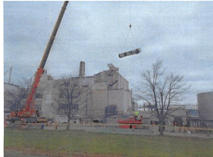
Removing VEC 36-inch duct from MPPB roof
