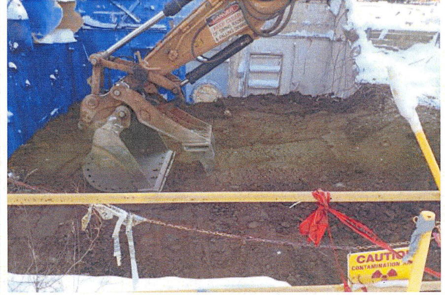
Below-grade Head-End Vent Blower Room after demolition and during backfilling
