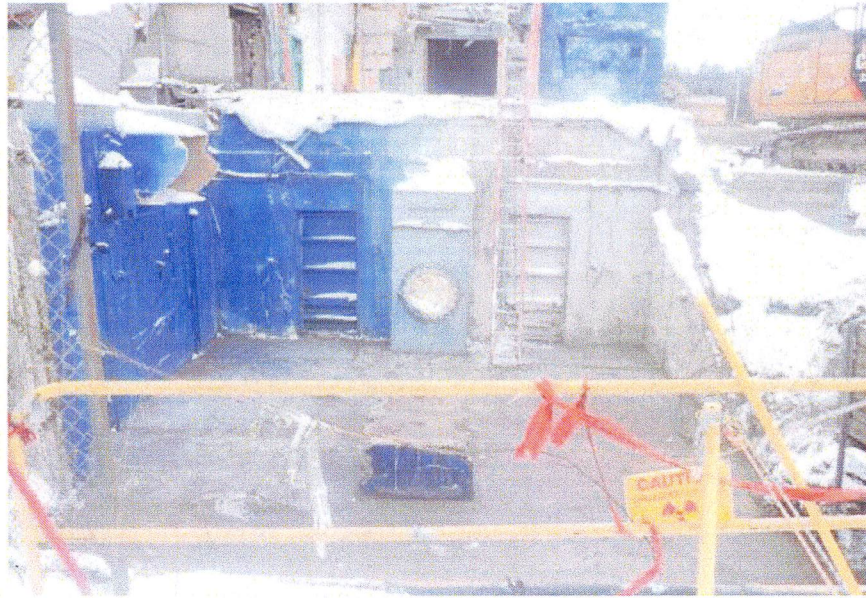
Below-grade Head-End Vent Blower Room after demolition and during backfilling
