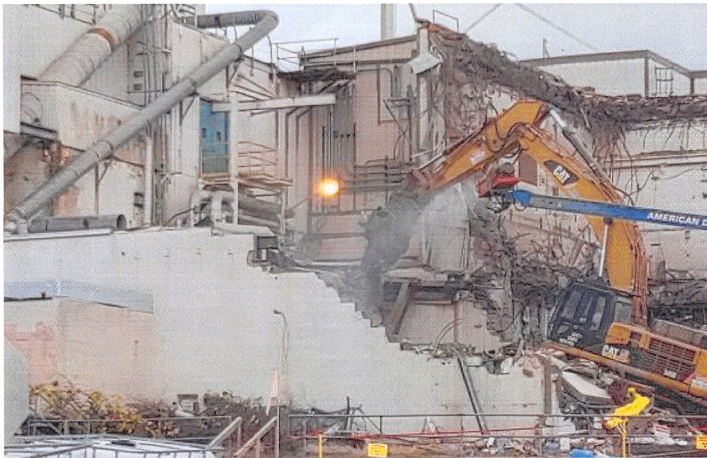
MSM Shop Demolition
