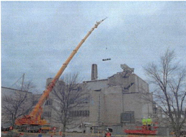
Removing VEC 36-inch duct from MPPB roof
