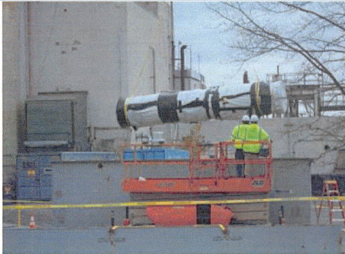
Removing VEC 36-inch duct from MPPB roof
