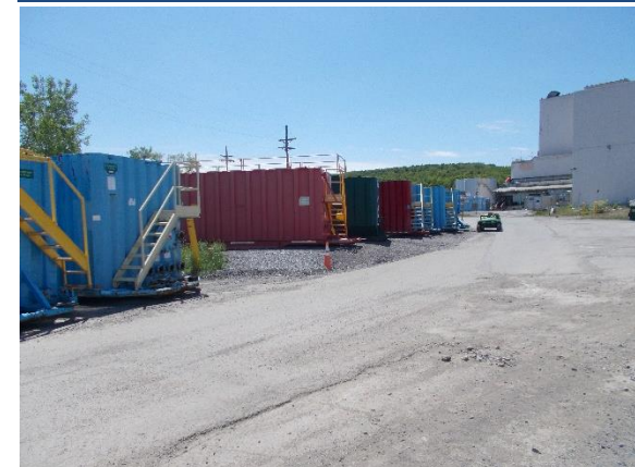
Water Management System construction
