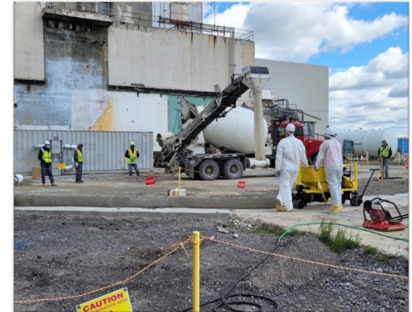
Constructing a berm
