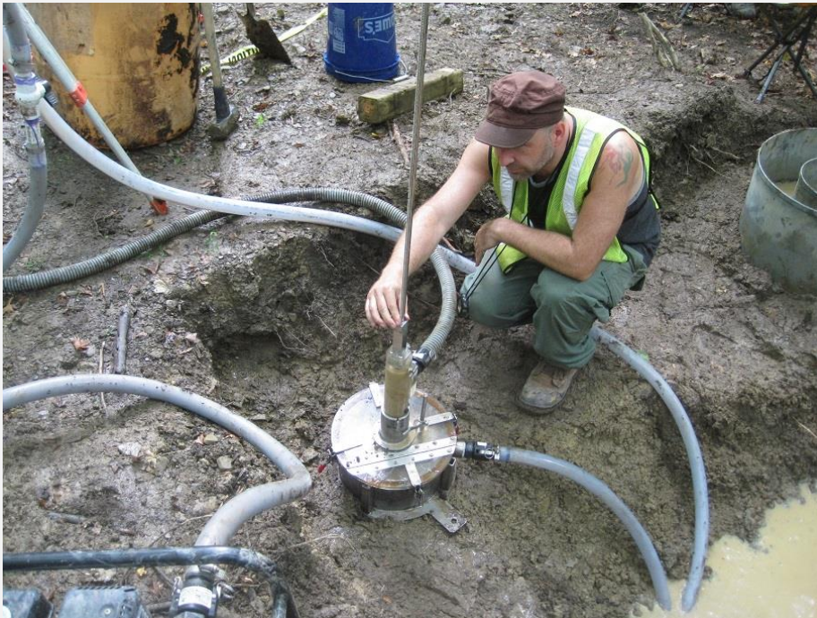
Jet testing in shallow pit
