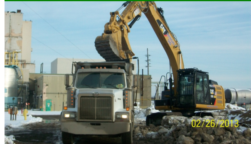
Waste load out of Old Warehouse foundations
