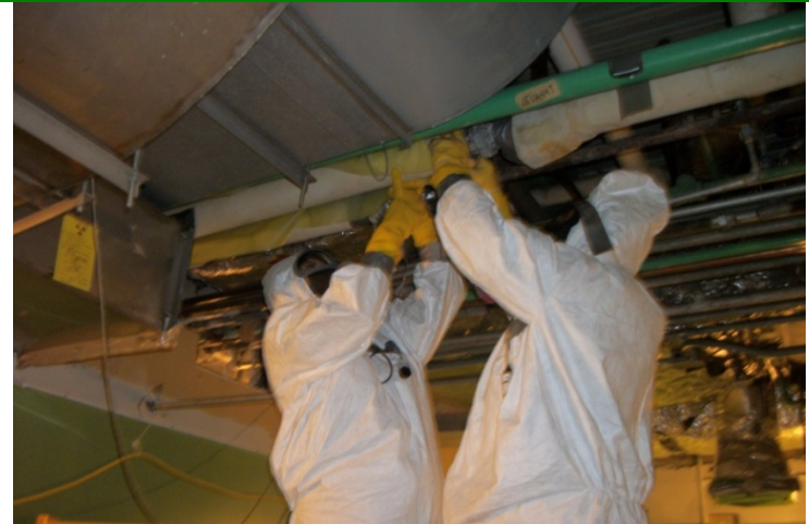
ACM Abatement in Analytical Aisle
