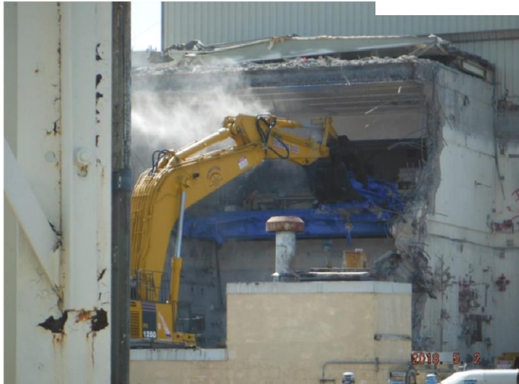
Process Crane Removal
