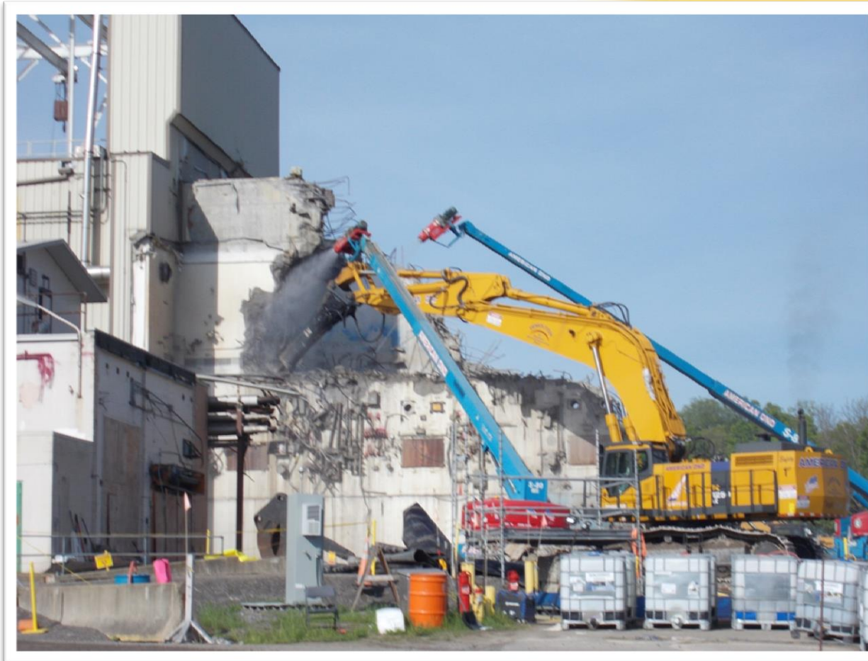
Vitrification Demolition (East Wall & Roof)
