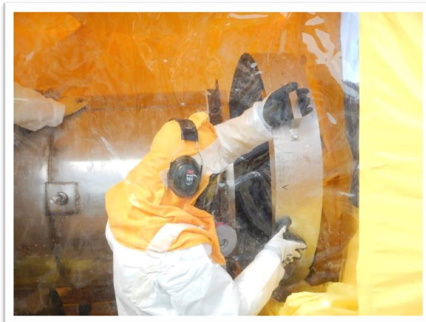
Preparing to cut 36-inch MPPB roof duct
