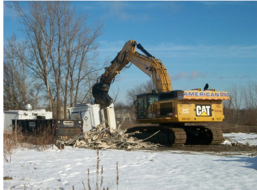
Hazardous Waste Locker Demolition
