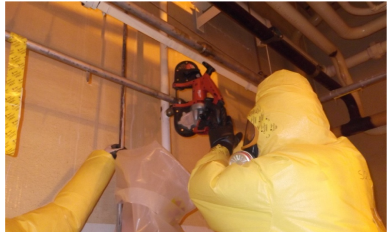
Chemical Piping Removal in LXA/COA
