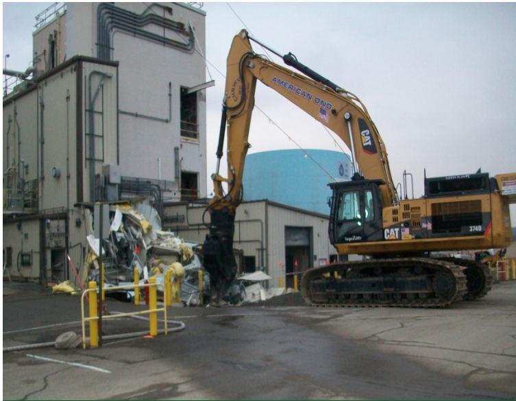
01-14 Building Demolition December 19, 2012 Step 1
