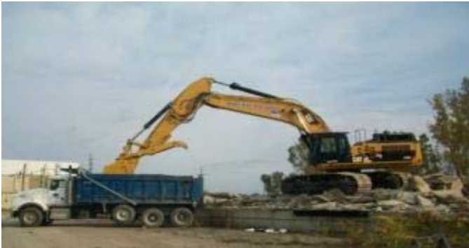
Waste Load Out of the Old Warehouse Pad
