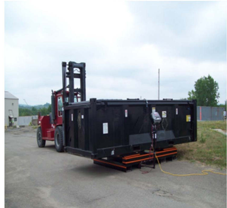
Preparing intermodals for demolition activities and loading of newly generated LLW
