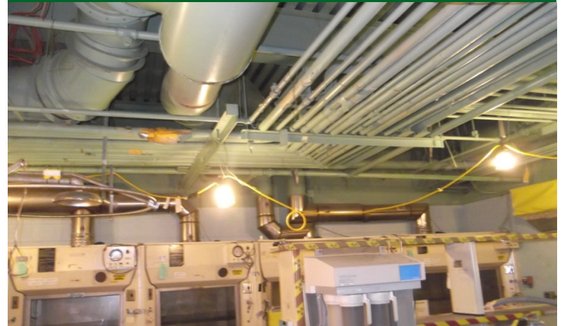
Radio-Chemical Lab Prepared for Asbestos Containing Material Removal
