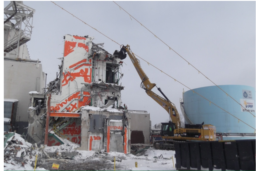
01-14 Building Demolition February 22, 2013 – Step 2
