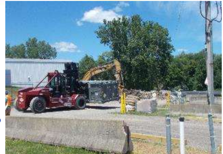
Workers load PTW soils for shipment on rail line
