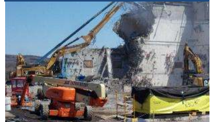
Vitrification Facility demolition
