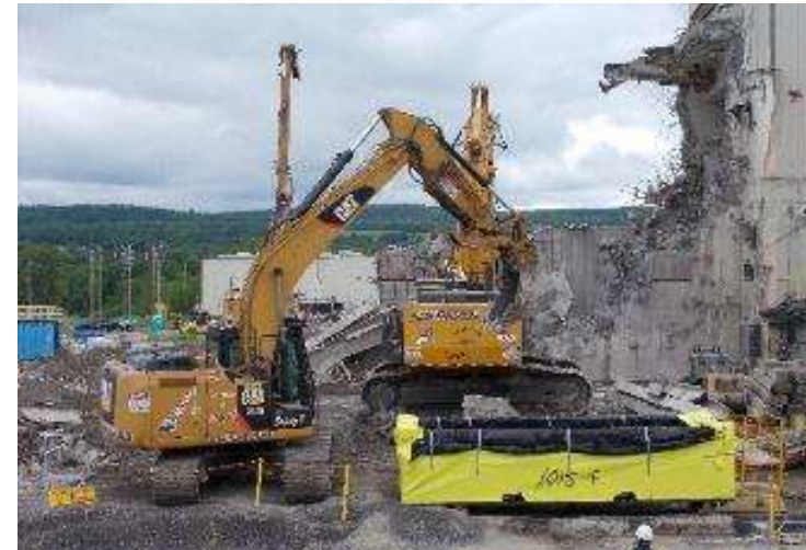
Waste loaded during Vitrification Facility demolition
