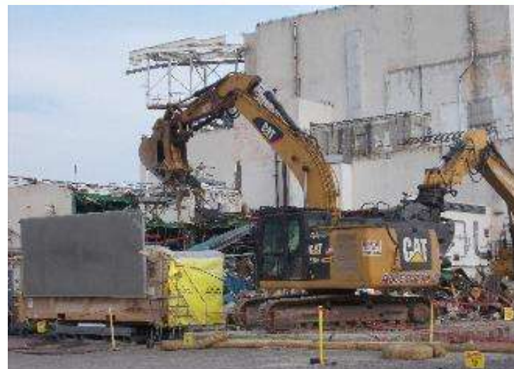
Waste being loaded into an intermodal during Utility Room demolition
