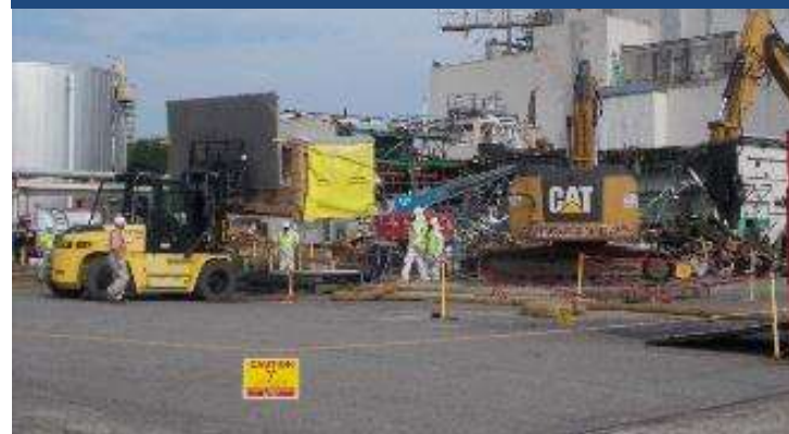
Waste being loaded into an intermodal during Utility Room demolition
