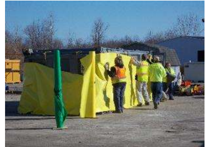
Workers prep a waste box for demolition debris
