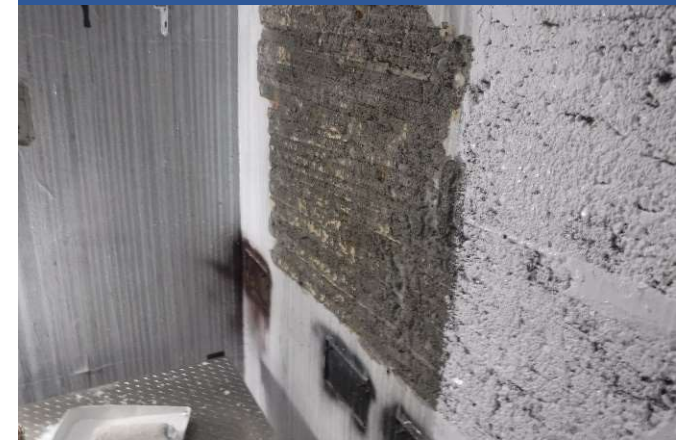
PPC-S wall 'scabbled' after using Nitrocision (October 2021)
