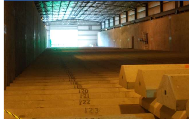
Inside Drum Cell (new roll-up door opening in background)
