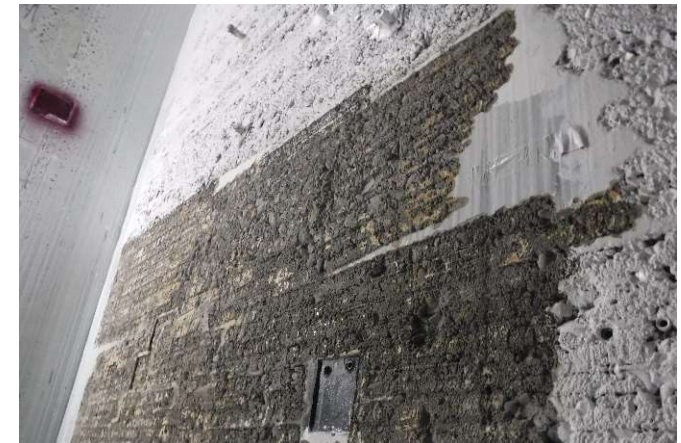
PPC-S wall 'scabbled' after using Nitrocision (October 2021)
