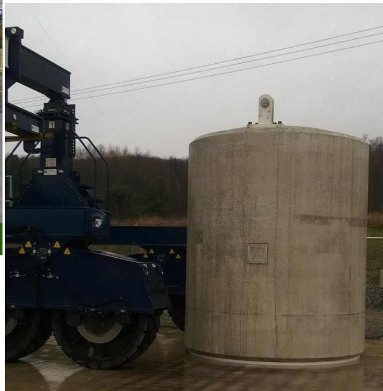
1 st Cask Placed on the Interim Storage Pad
