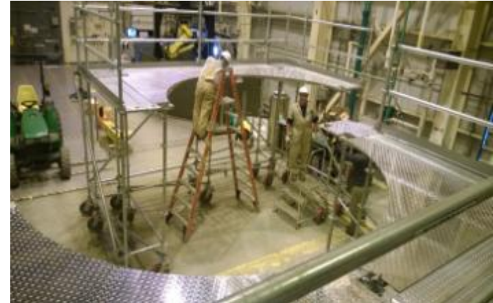
Erected Cask Preparations Platform
