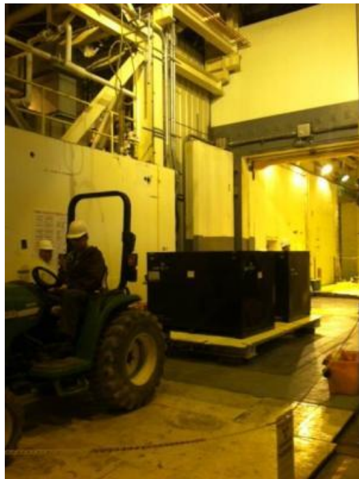
Equipment Decontamination Room (EDR) Waste Removal for Shield Door Repair
