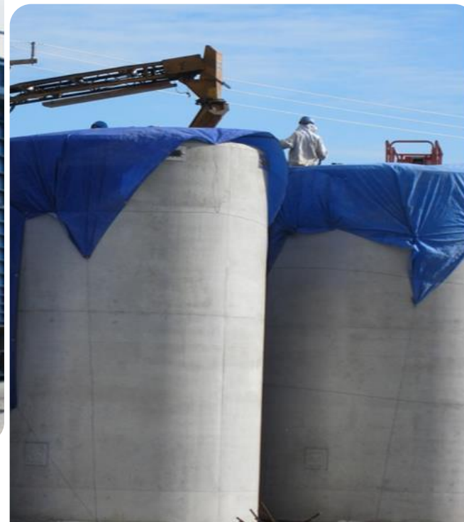
Vertical Storage Casks Fabricated on Site
