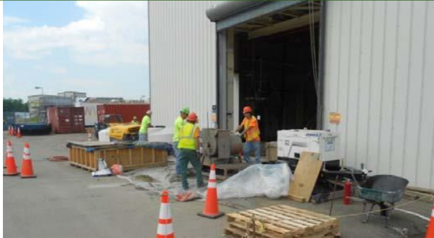
Installed LIF Floor Plating
