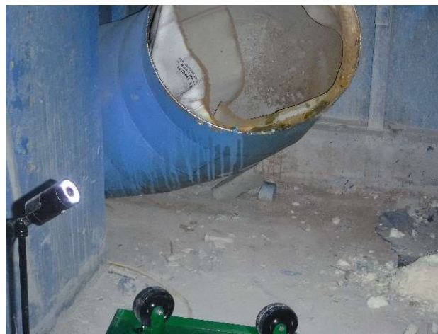
Section of cut vent duct in VWR
