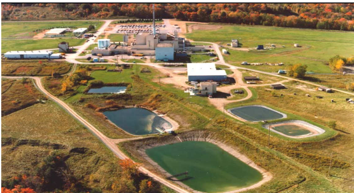
Figure ES-4. The Plant During the Early Years (The lagoons appear in the foreground. The Process Building can be seen in the background.)
