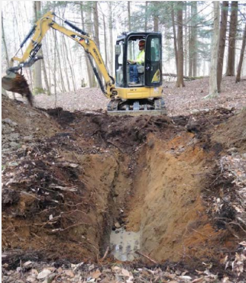
Trench excavation in progress (location chosen with assistance of GPR survey)
