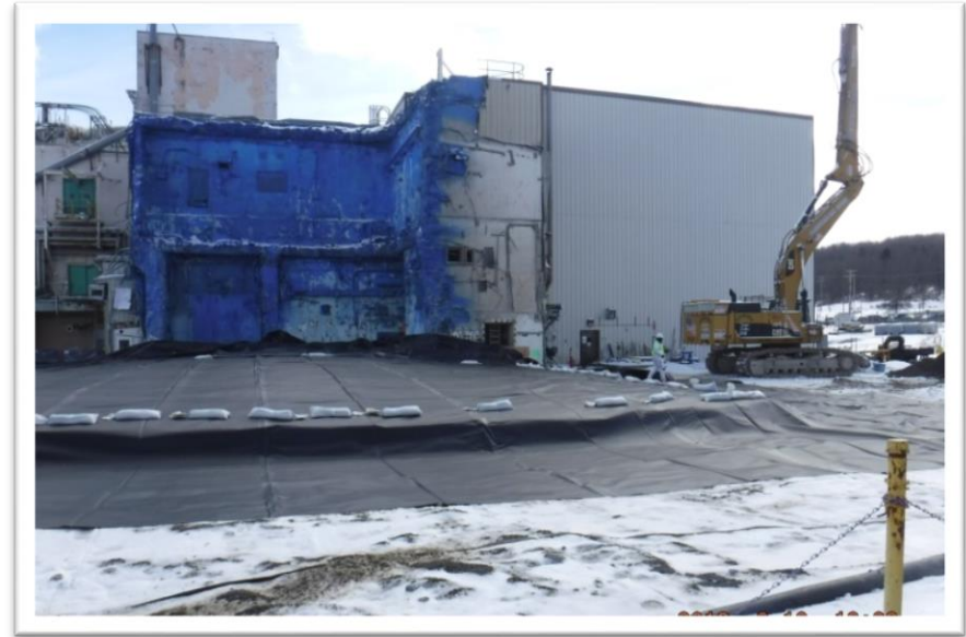
Former location of Vitrification Facility (Main Plant Process Building in background)
