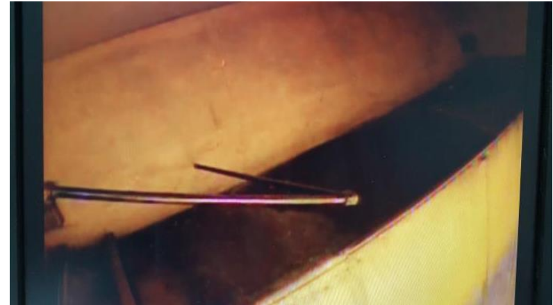
South Ledge Before Decontamination
