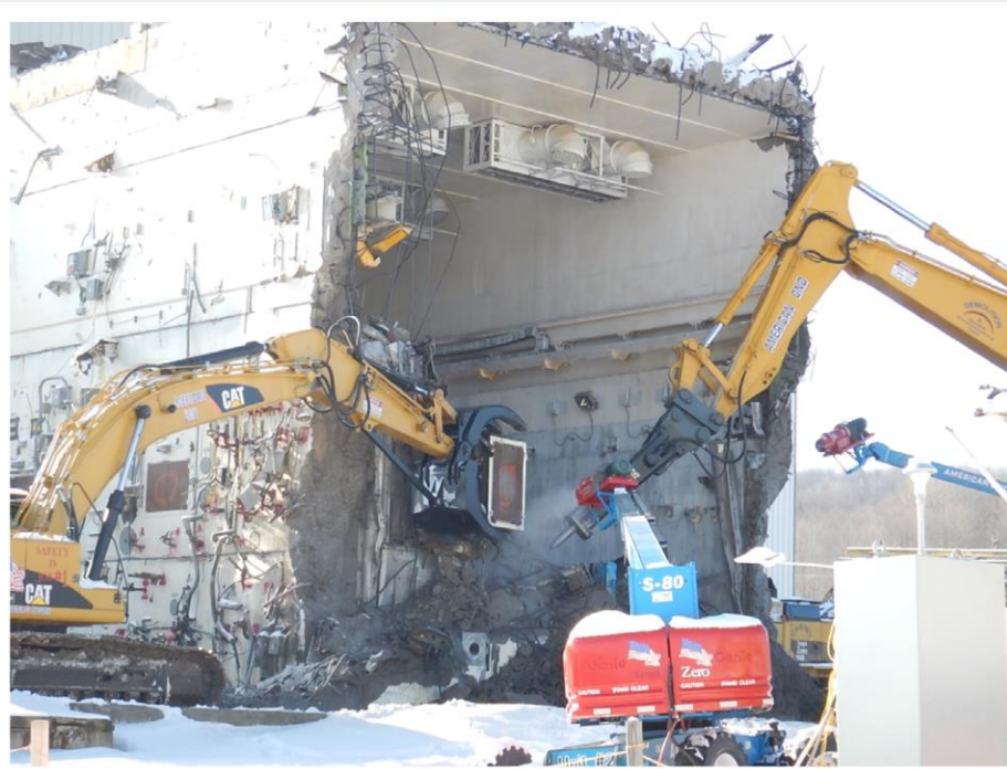
Removal of second shield window from the Vitrification Facility January 19, 2018
