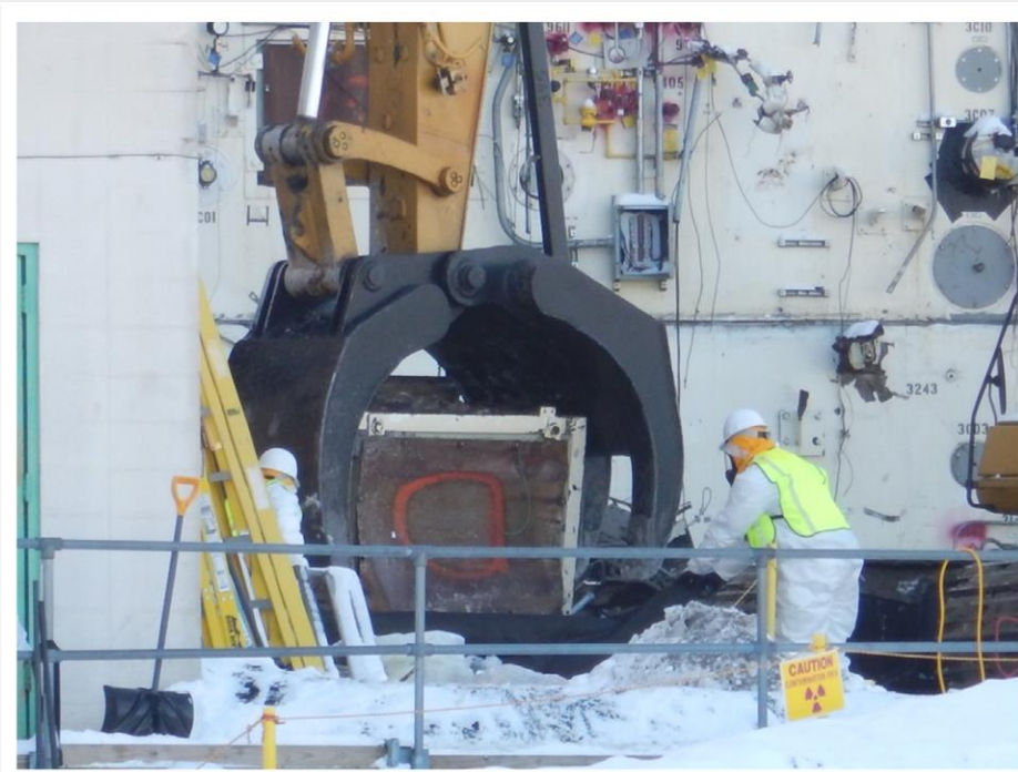
Removal of second shield window from the Vitrification Facility January 19, 2018
