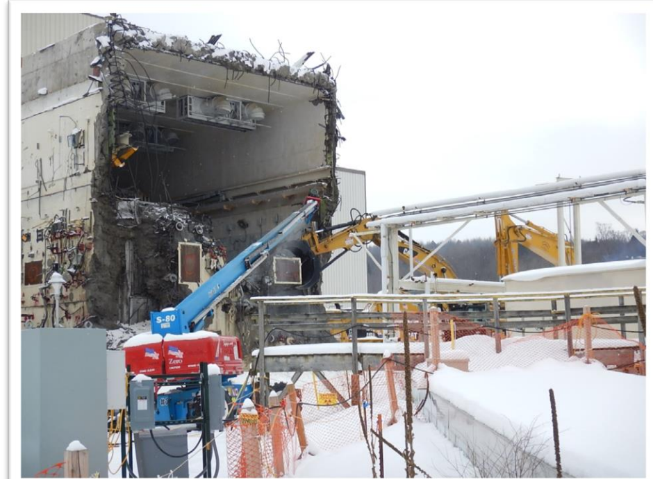
Removal of first shield window from the Vitrification Facility January 18, 2018
