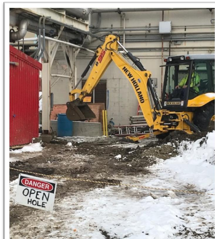
Work being performed on the site's fire loop
