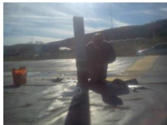
NDA Inspection and Repair
