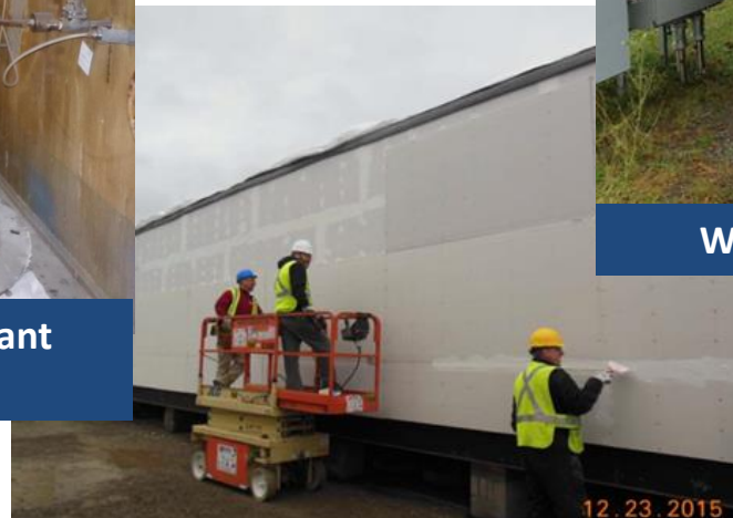
10-Plex Office Installation
