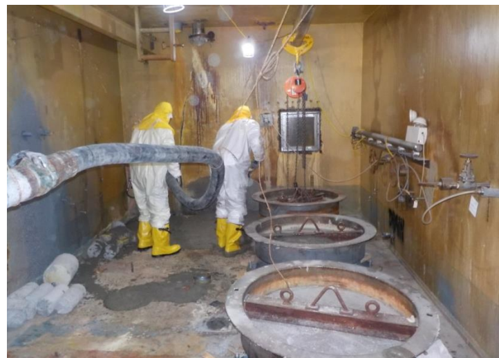
OGBR Floor and Niche Grouting
