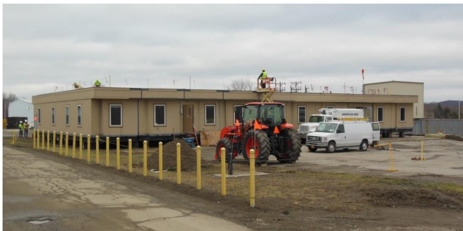
10-Plex Office Complex Set-up Underway
