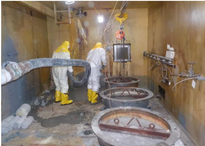
Grouting Activities in the Main Plant Process Building (MPPB)
