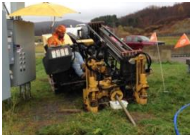
Water Line Installation
