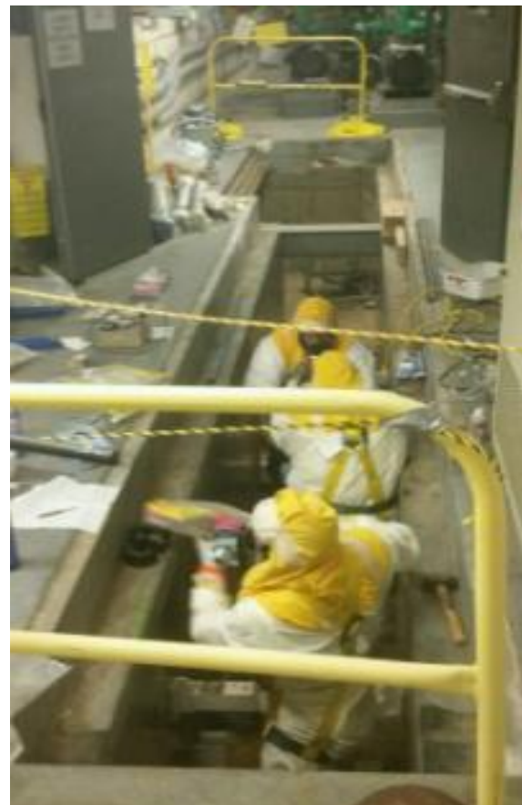
High-Level Waste Trench Pipe Removal
