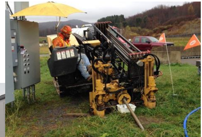
Water Line Directional Boring
