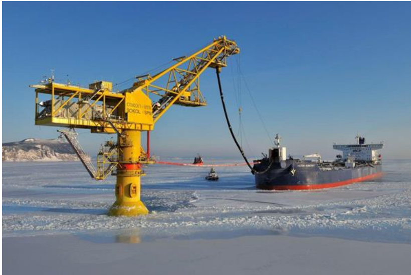
Figure 4. Loading at DeKastri Single Point Mooring Loading Platform in light ice. (Photo: Sakhalin 1 Project)
