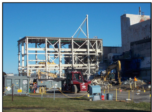
Demolition of the Load-In/Load-Out (LILO) facility
