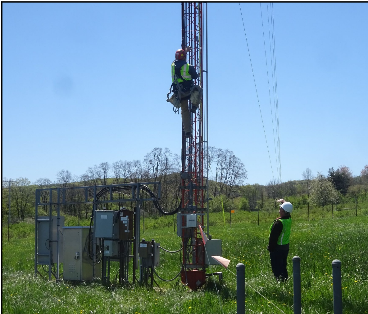
On-site meteorological monitoring tower undergoing inspection with oversight by the full-time on-site meteorological monitoring engineer
