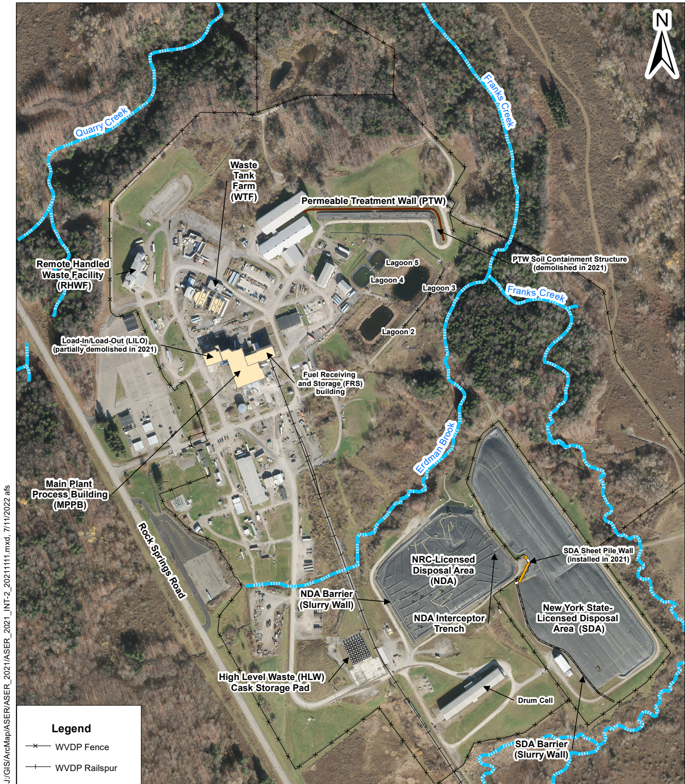
FIGURE INT-2 Aerial Photo of the West Valley Demonstration Project
