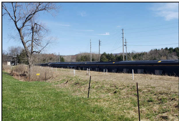
PTW soil containment structure (covered with a black tarp)
