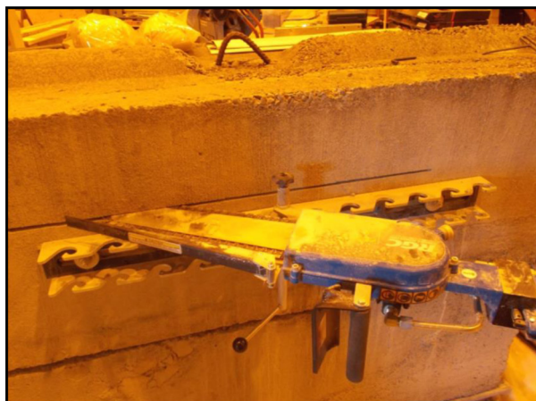
Diamond wire saw (used with misting)
