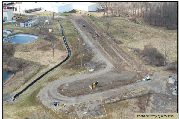
PTW area after removal of the soil containment structure
