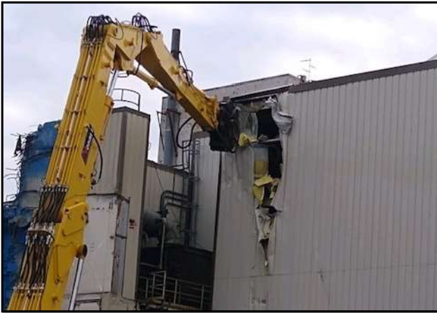
First stages of Load-In/Load-Out (LILO) demolition
