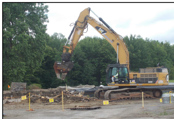
Demolition and removal of PTW soil containment structure
