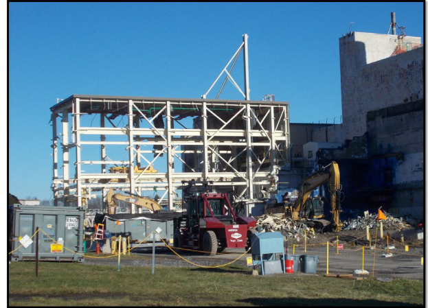
LILO demolition status at the end of December 2021
